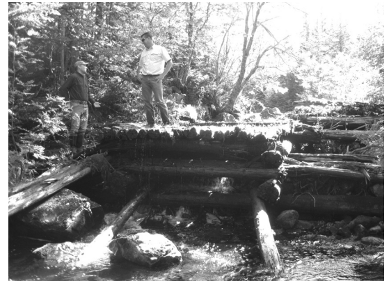
Figure 14. Remnant splash dam near the headwaters of Intervale Brook. This dam continues to be a barrier to fish passage and is scheduled for removal in Fall 2013. Photo Credit: Merry Gallagher.
