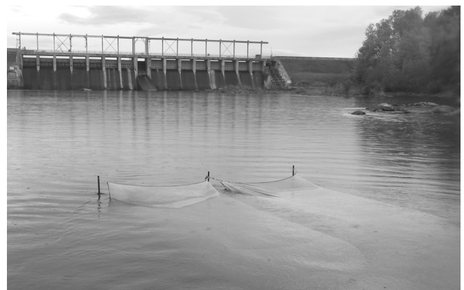
Figure 24. Deployed smelt drift nets below Brassua Lake Dam.
