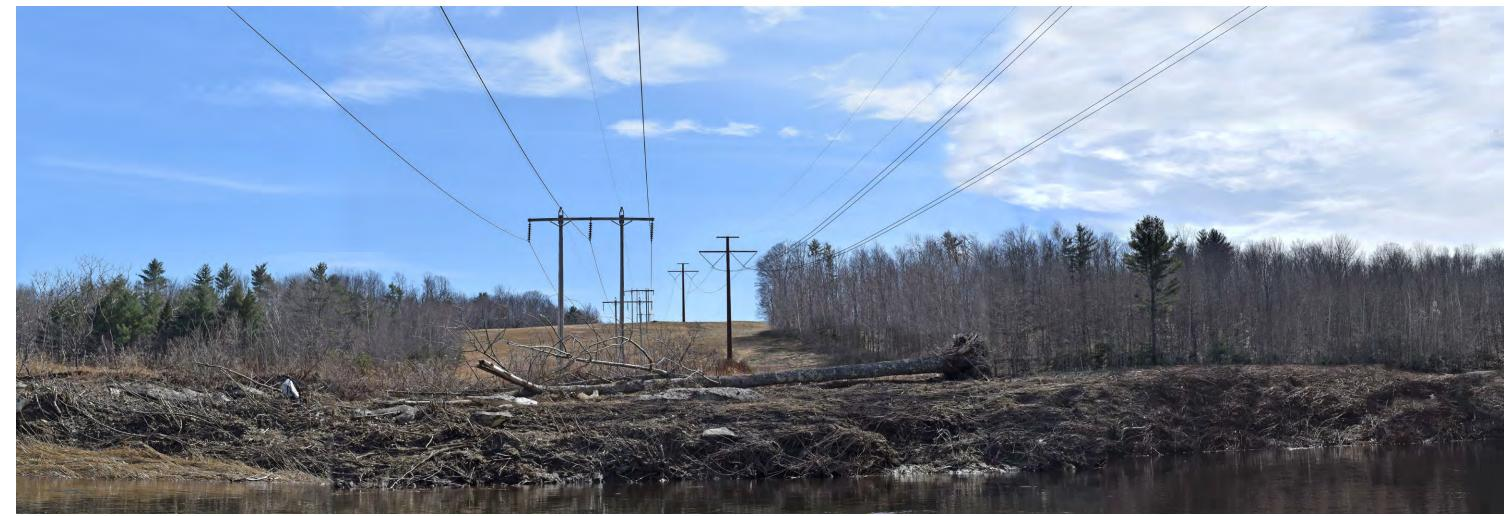
**Proposed Conditions:** Panoramic view looking south to west from the Sandy River in Farmington toward the proposed co-located HVDC transmission line. The existing 225' wide cleared corridor will be widened by 75' on the western side to accommodate the proposed HVDC transmission line. Two proposed HVDC structures and conductors will be visible at distances of 825 to 1,600 feet from this viewpoint.
