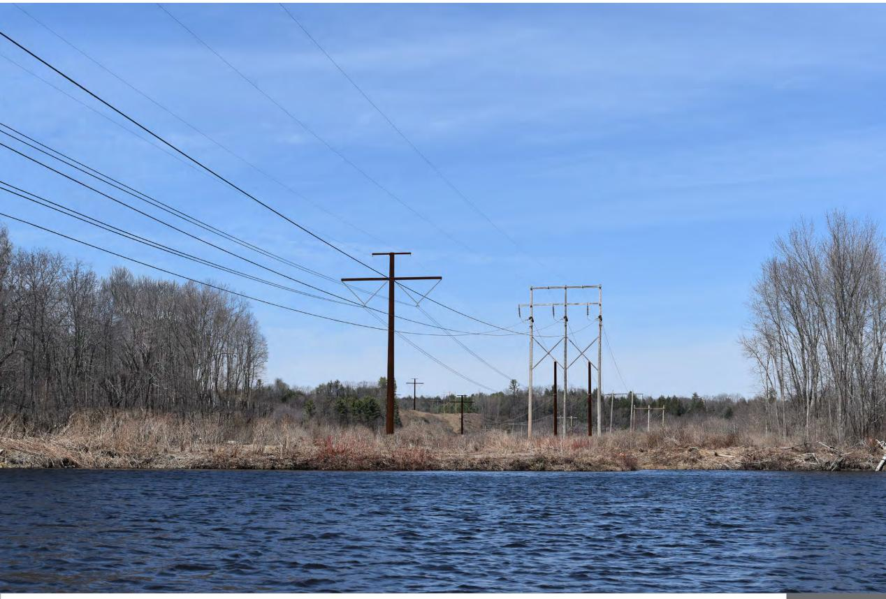
**Proposed Conditions:** Normal view looking north from the Carrabassett River in Anson toward the proposed co-located HVDC transmission line. The existing 225' wide cleared corridor will be widened by 75' on the western side to accommodate the proposed HVDC transmission line. Five proposed HVDC structures and conductors will be visible at distances of 540 feet to 3,160 feet from this viewpoint.
