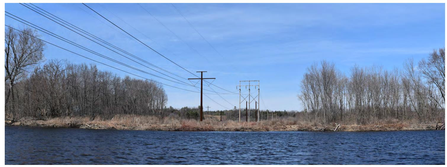
**Proposed Conditions:** Panoramic view looking north to northwest from the Carrabassett River in Anson toward the proposed co-located HVDC transmission line. The existing 225' wide cleared corridor will be widened by 75' on the western side to accommodate the proposed HVDC transmission line. Five proposed HVDC structures and conductors will be visible at distances of 540 feet to 3,160 feet from this viewpoint.
