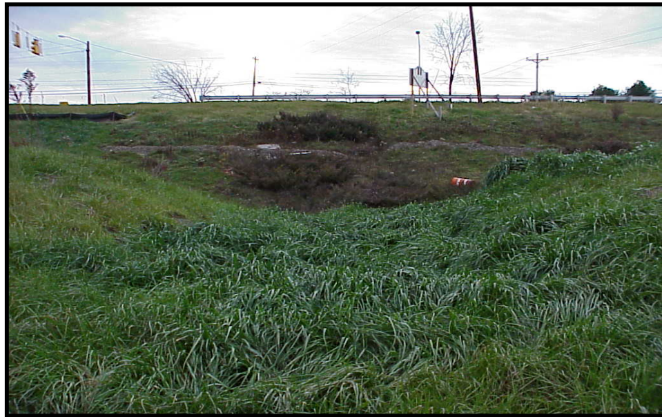
A well-stabilized vegetated swale shows little sign of erosive velocities or flows.
