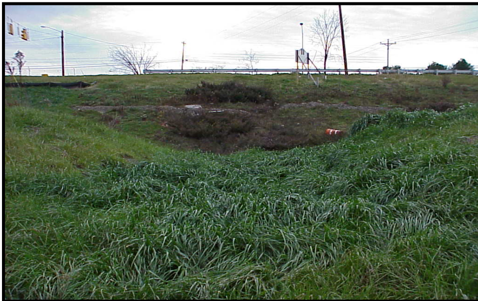
A well-stabilized vegetated swale shows little sign of erosive velocities or flows.
