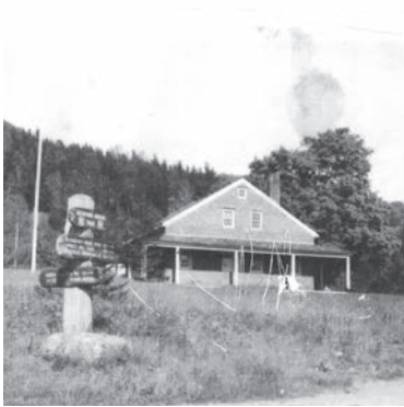
Brickett Place farmhouse Image courtesy of White Mountains Interpretive Association
