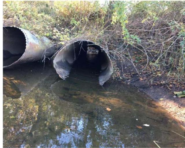
Willow Brook Culvert - Highest priority for replacement in study
