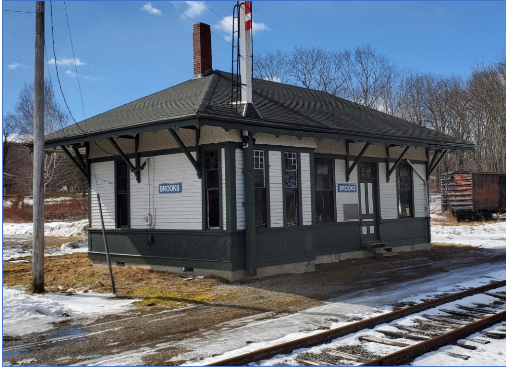
Figure 5: Brooks Rail Station, National Historic Register 2009
