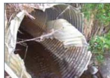
damaged culvert
