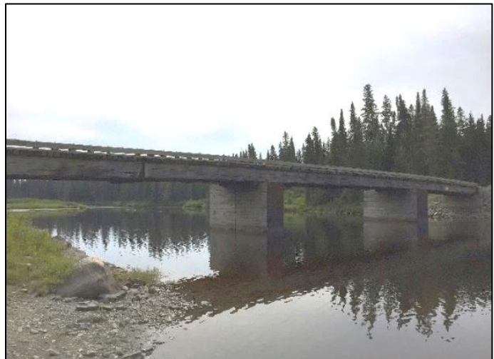
Reburbished Henderson bridge over the Allagash River, BPL Northern Region
