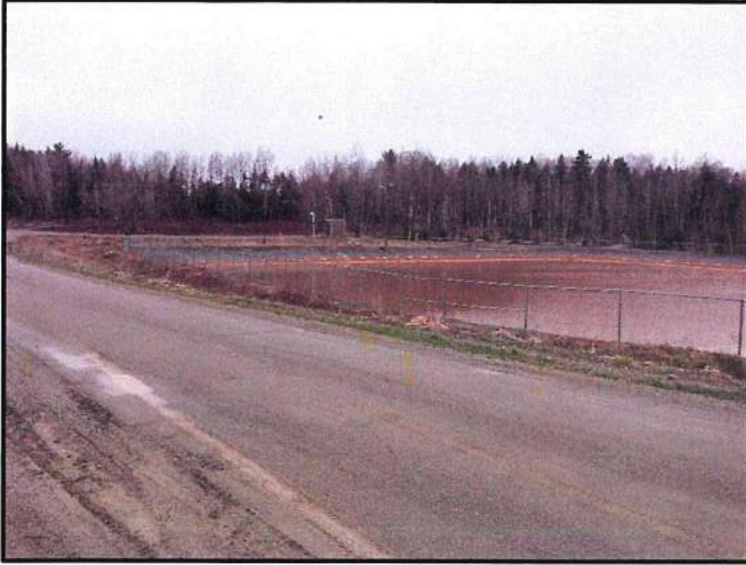
Dolby III Leachate Pond.
