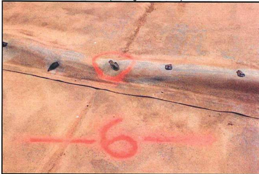
Repair (Damage Location 6)
