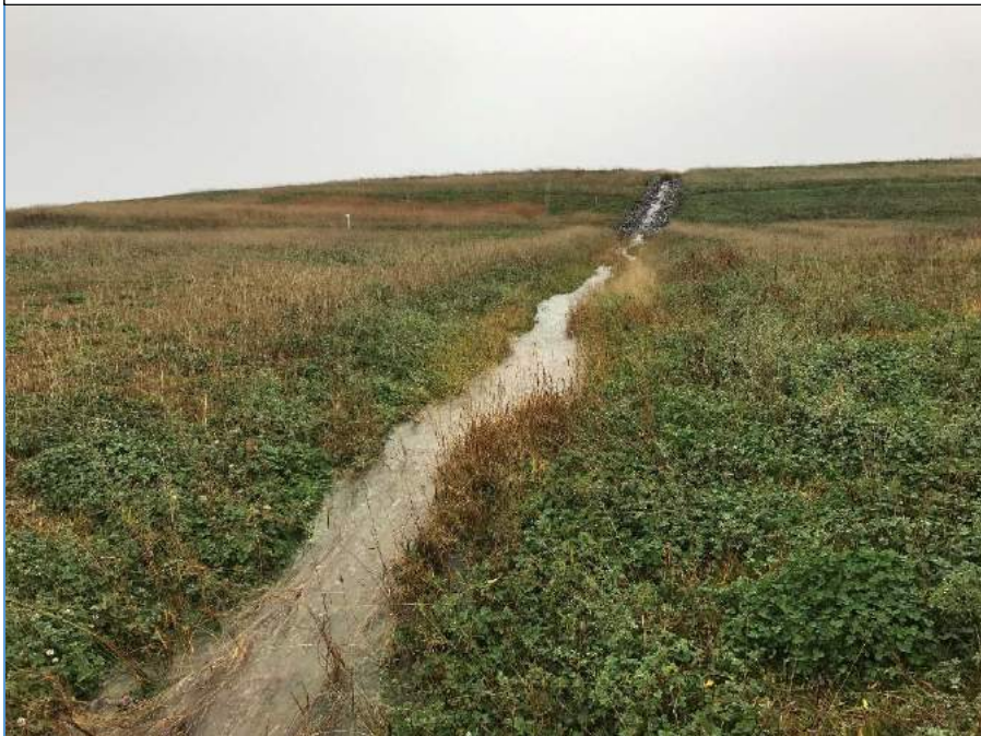
DOLBY III GRASS CHANNEL ON PHASE I COVER UPGRADE
