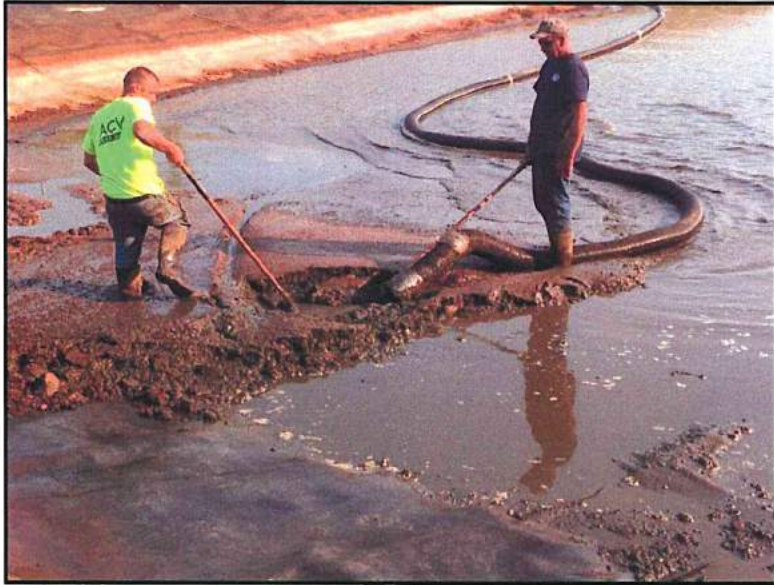
Leachate Pond Liner Cleaning
