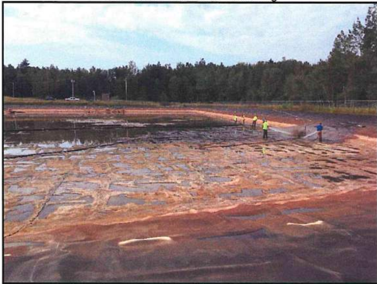
Leachate Pond Liner Cleaning
