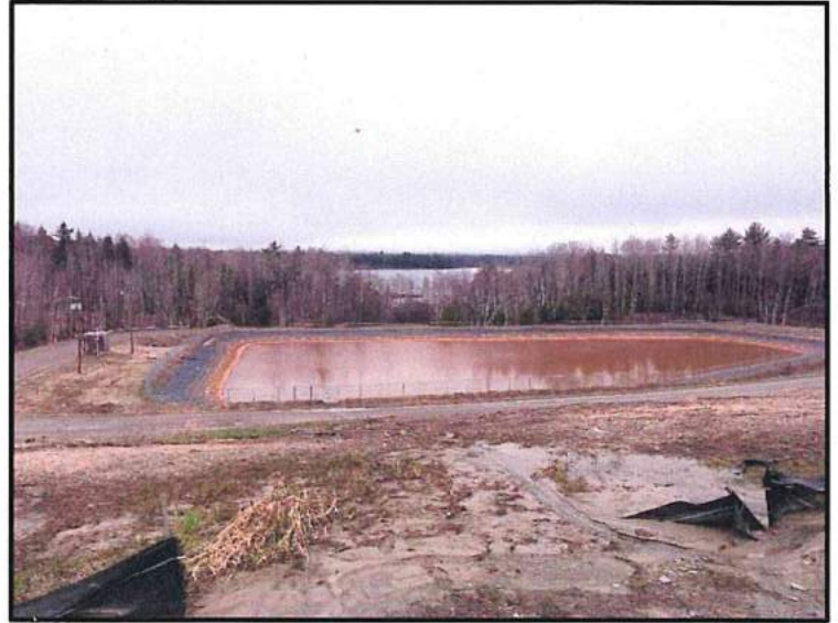
Dolby III Leachate Pond.
