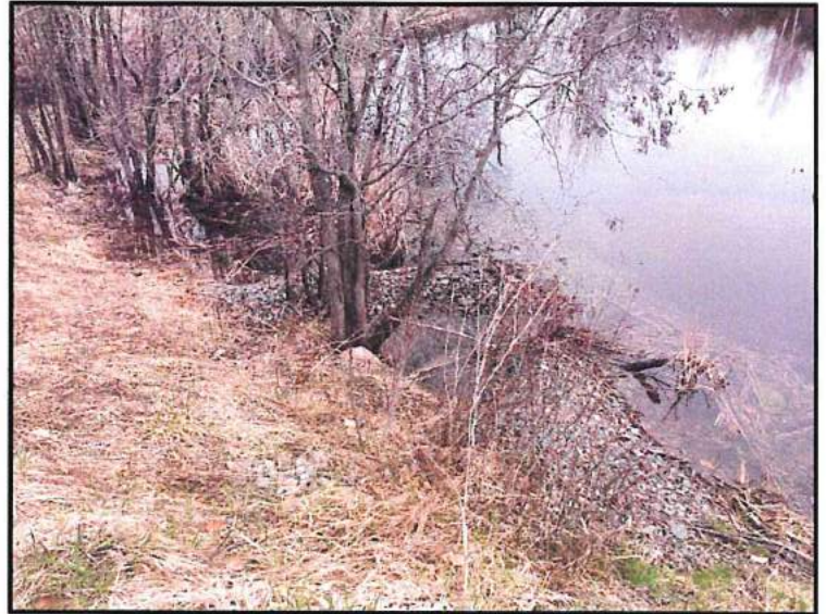
Southwest sediment pond outlet.
