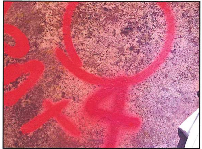
Dent (Damage Location 4)
