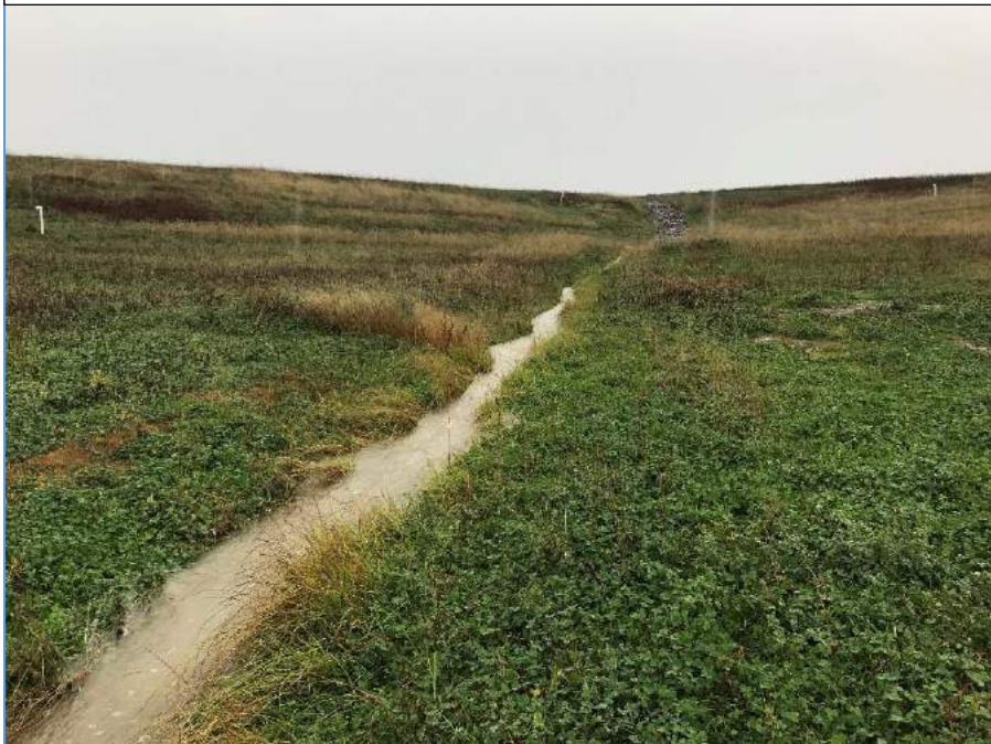
GRASS-LINED DITCH ON PHASE I COVER UPGRADE AREA
