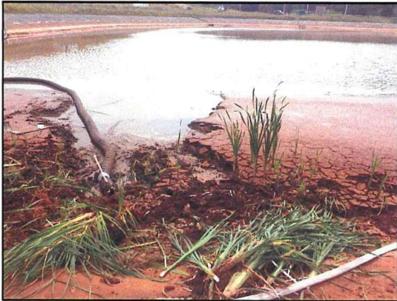
Leachate Pond Liner Cleaning
