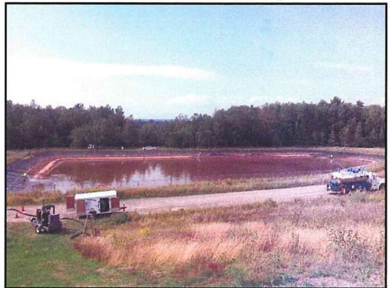
Leachate Pond Liner Cleaning
