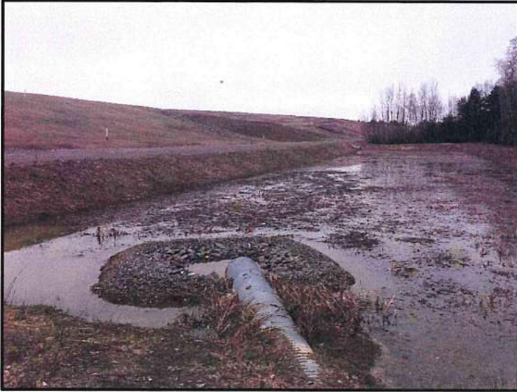
Northwest sediment basin.
