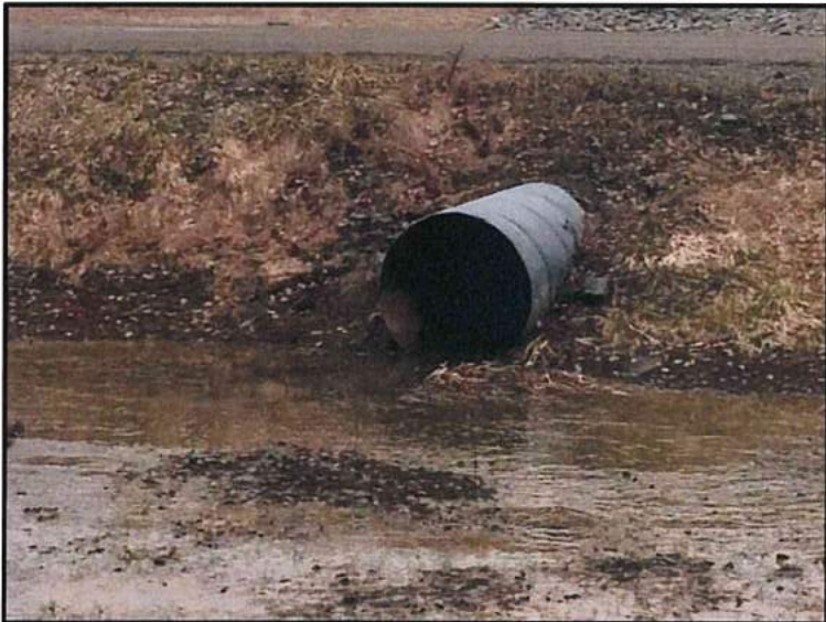
Northwest sediment basin inlet pipe.
