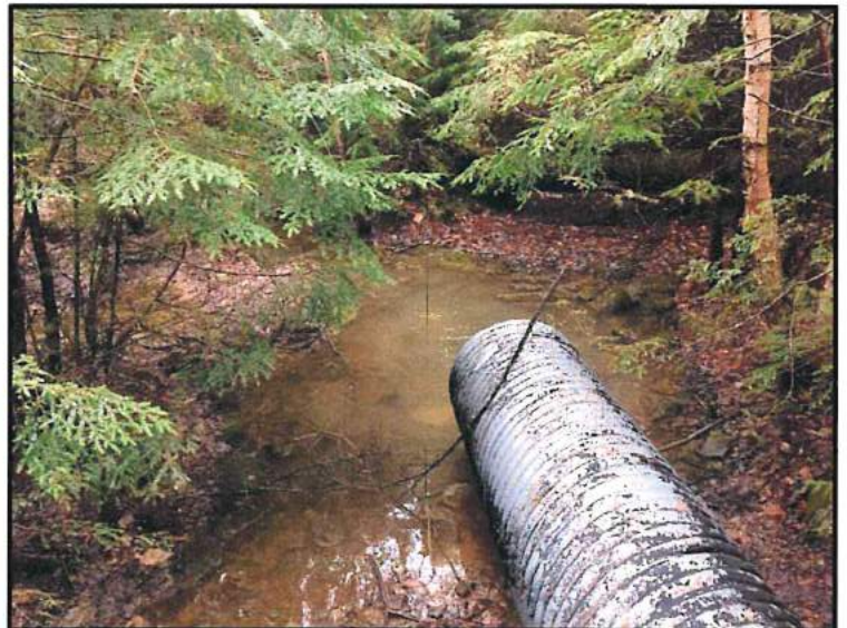
Northwest sediment basin outlet pipe.
