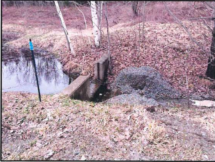
West sediment pond outlet.
