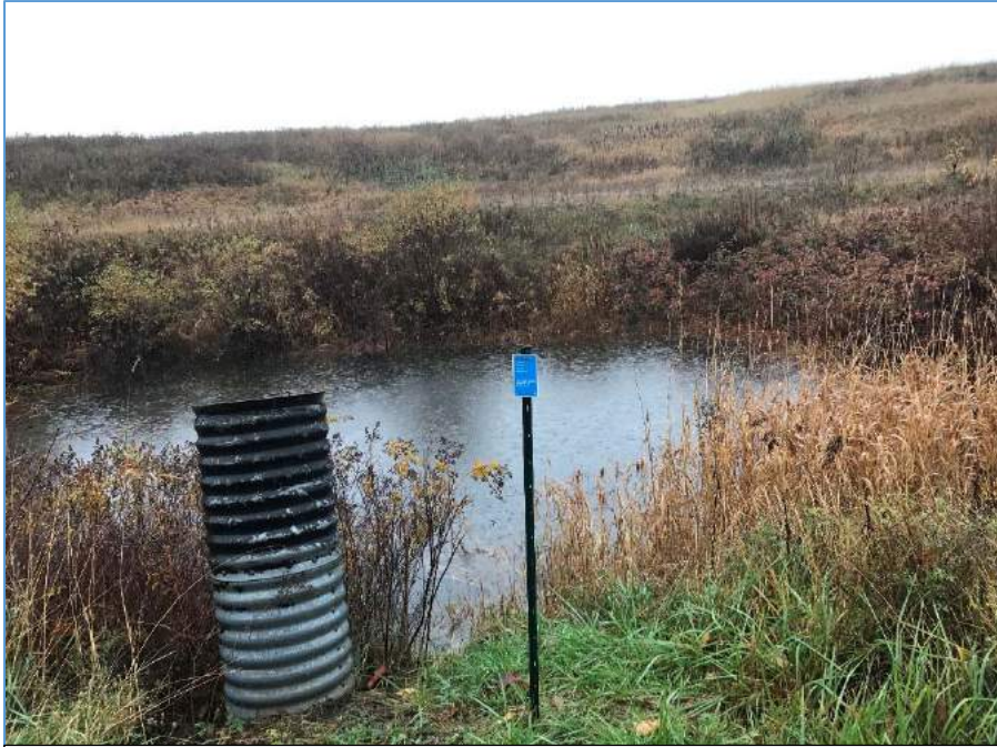
DOLBY II LEACHATE POND – EAST SIDE
