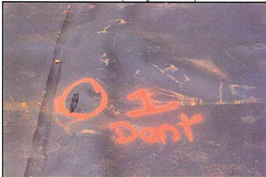
Repair (Damage Location 1)
