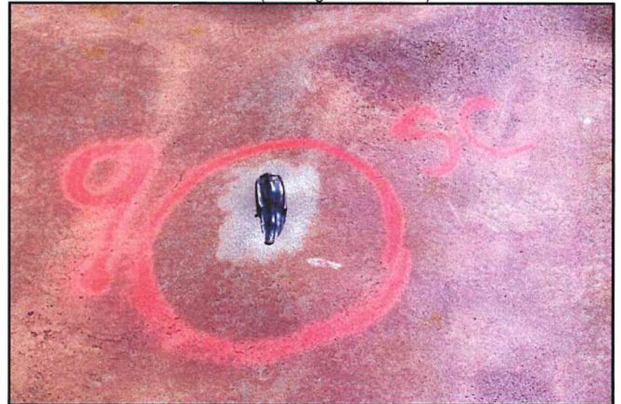
Repair (Damage Location 9)
