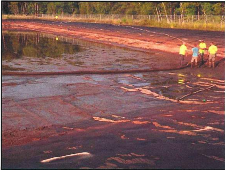
Leachate Pond Liner Cleaning
