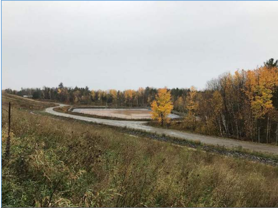
DOLBY III LANDFILL WITH LEACHATE POND IN BACKGROUND
