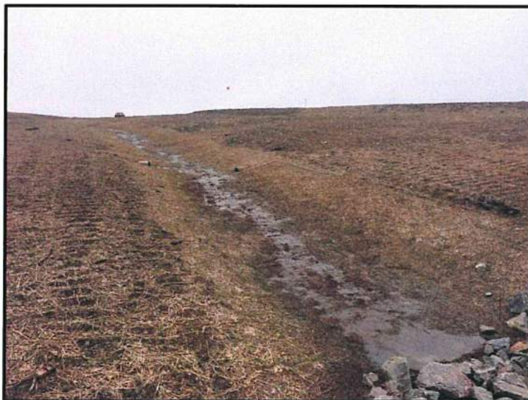
Grass ditch Phase I cover upgrade area.
