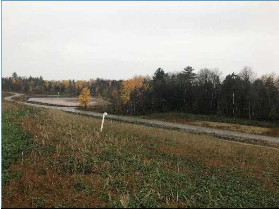
DOLBY III WITH LEACHATE POND AND NORTHEAST SEDIMENT POND IN BACKGROUND
