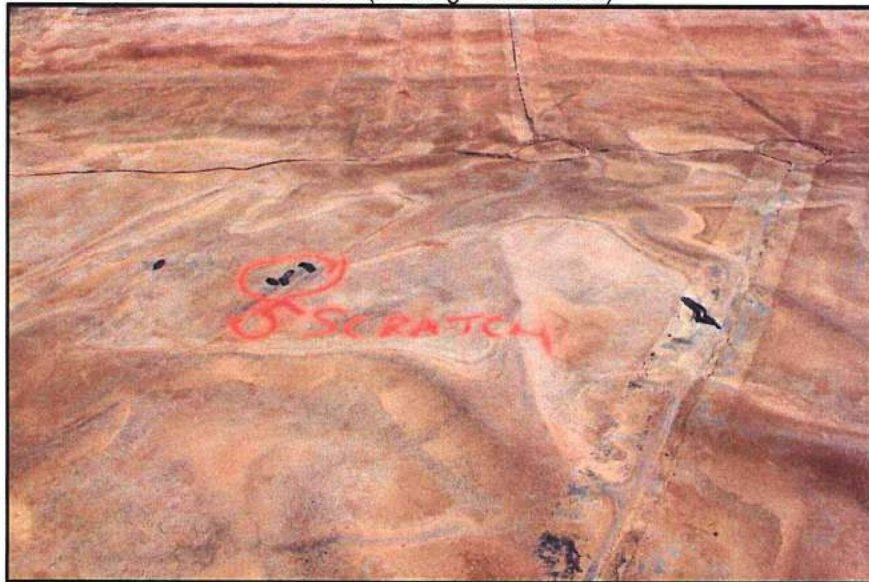
Repair (Damage Location 5)
