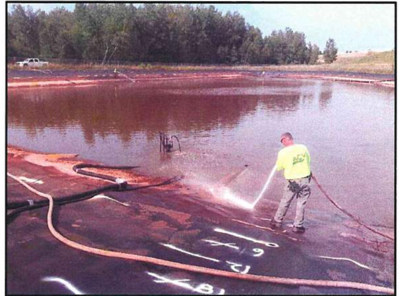
Leachate Pond Liner Cleaning
