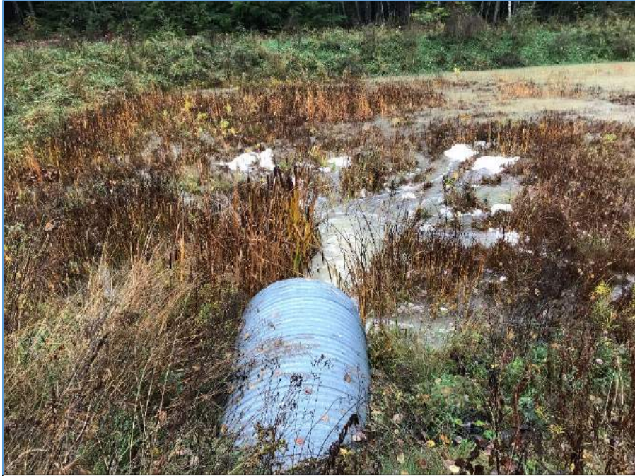
DOLBY III CULVERT INLET TO NORTHEAST SEDIMENT POND
