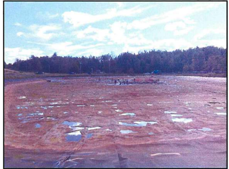
Leachate Pond Liner Cleaning
