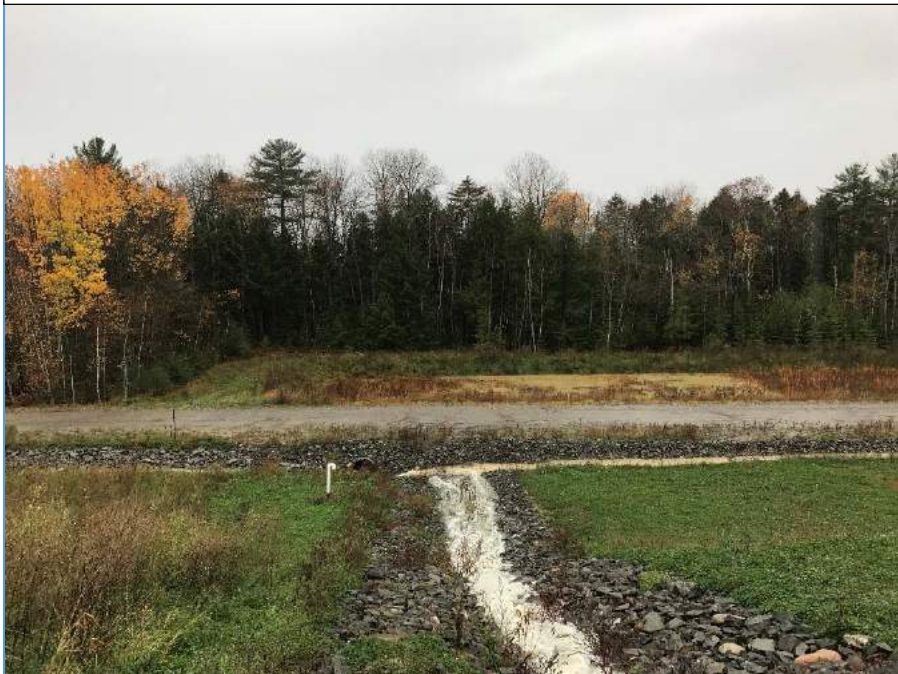
DOLBY III LANDFILL WITH NORTHWEST SEDIMENT POND IN BACKGROUND
