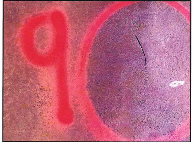
Scratch (Damage Location 9)
