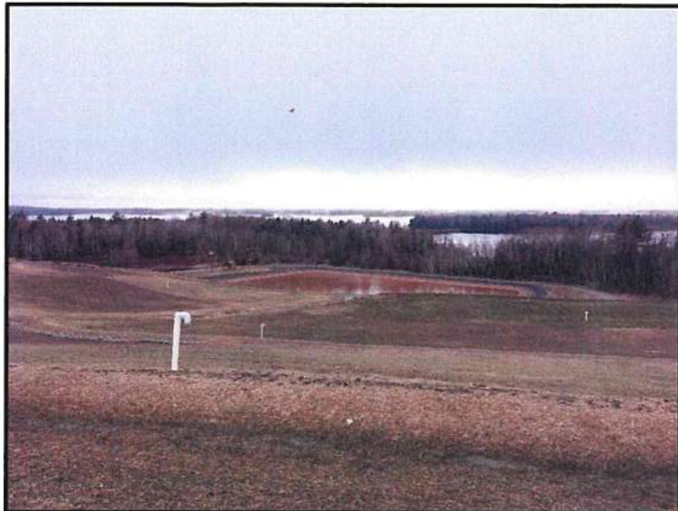
Leachate pond from Phase I cover upgrade area.
