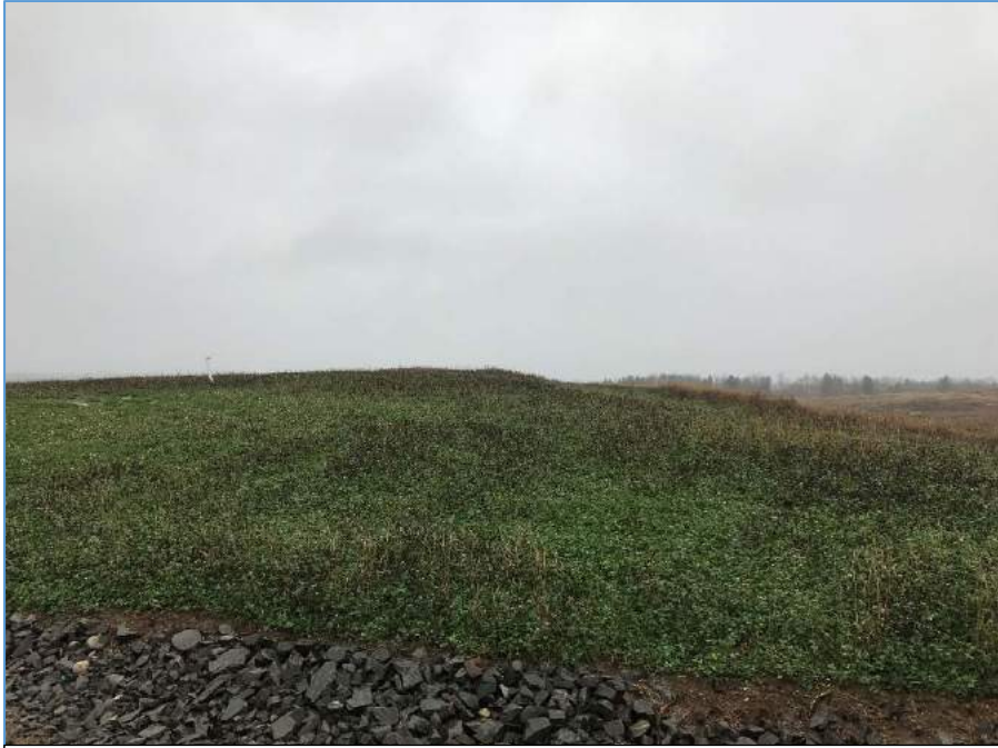
DOLBY III TOP OF PHASE I COVER UPGRADE AREA
