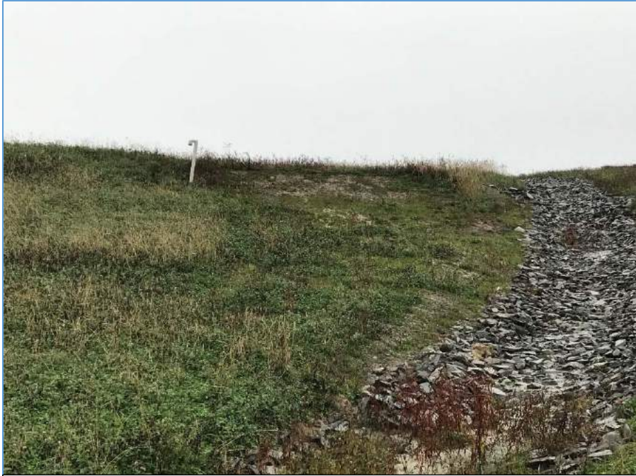
DOLBY III AREA OF SOIL EROSION AT TOP OF SOUTHERN-MOST DOWNSPOUT ON PHASE I COVER UPGRADE AREA
