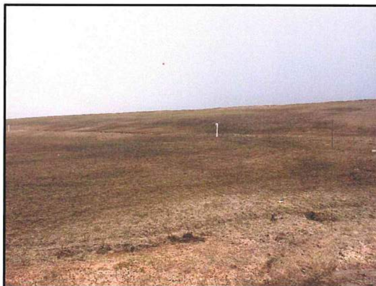
Phase I cover upgrade area.
