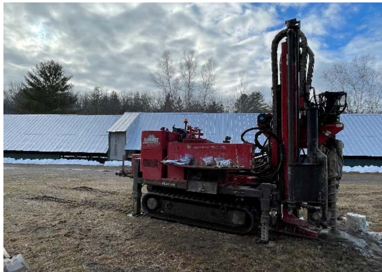
Drilling of Test Boring B-2
