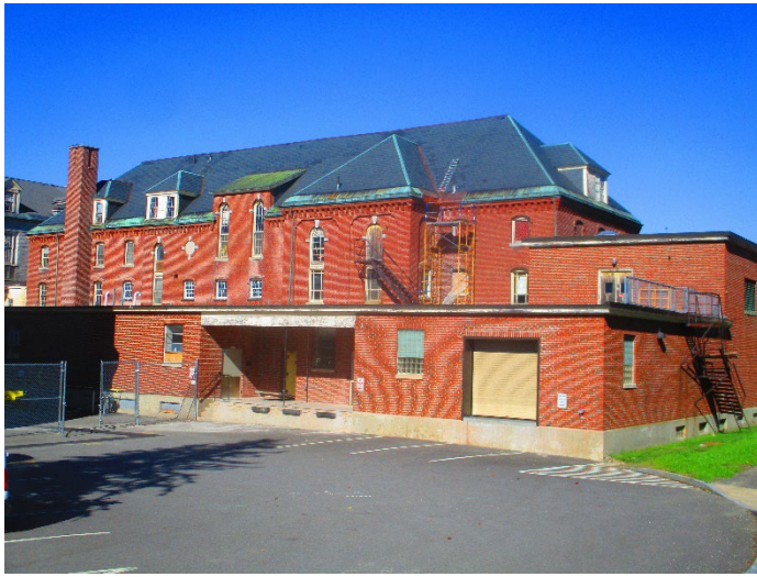
Photo 1: Exterior view of the Central Building facing North.
