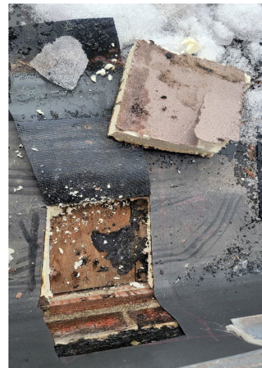
Photo 6: (12/21/2022): Typical roof cut.
