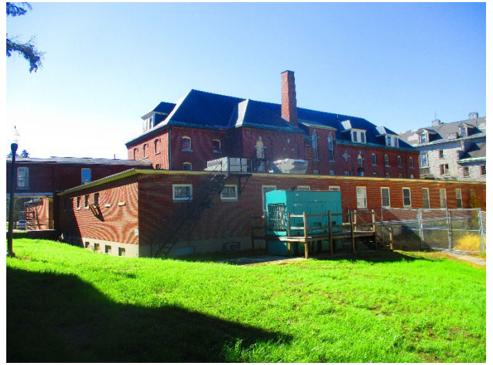
Photo 2: Exterior view of the Central Building facing South.
