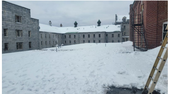
Photo 4 (12/21/2022): Roof Area A, conditions at time of assessment.
