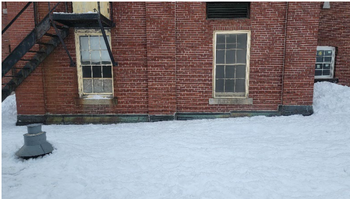
Photo 5 (12/21/2022): Roof Area B, conditions at time of assessment.
