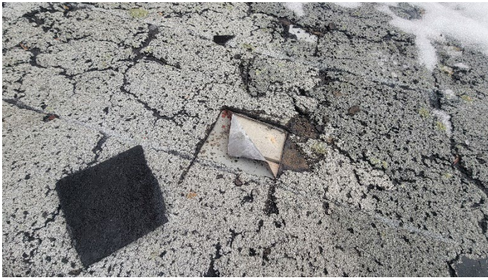
Photo 1 (March 9, 2023): ACM rolled asphalt roofing (sample set EW-01) present on Roof Area D2.
