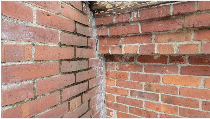
Photo 3 (March 9, 2023): ACM caulking (sample set EW-03) present at the interface of the elevated walkway and the Elkins Building.
