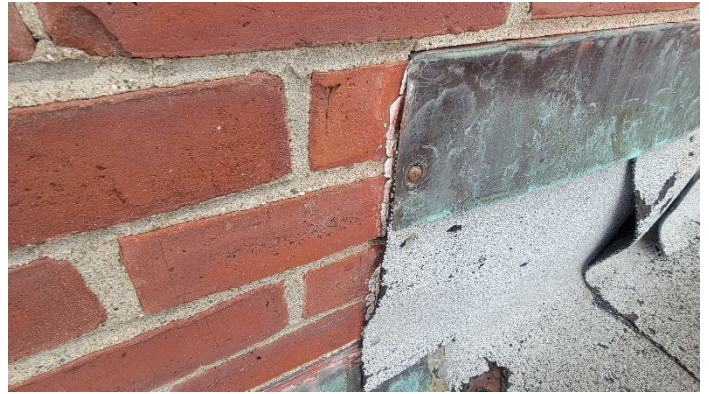
Photo 4 (March 9, 2023): ACM caulking (sample set EW-04) located at the flashing/building interface.
