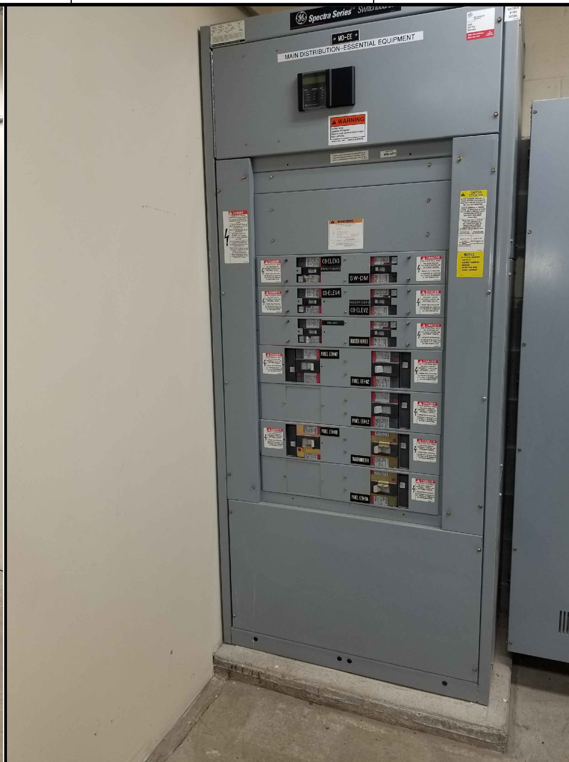
E4 PHOTO #3 - MD-EE (EXISTING) DO NOT SCALE
