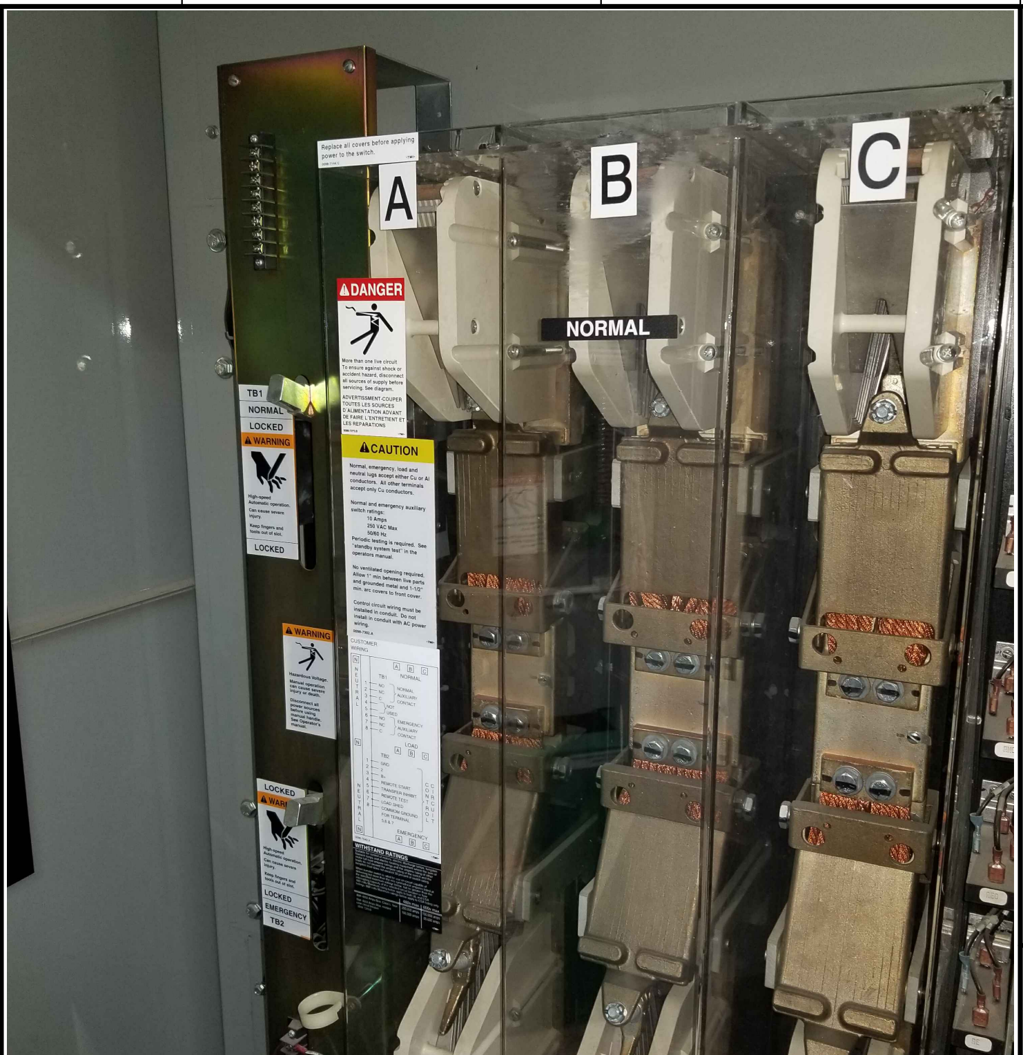
E8 PHOTO #5 - ATS - EE (EXISTING INTERIOR UPPER) DO NOT SCALE
