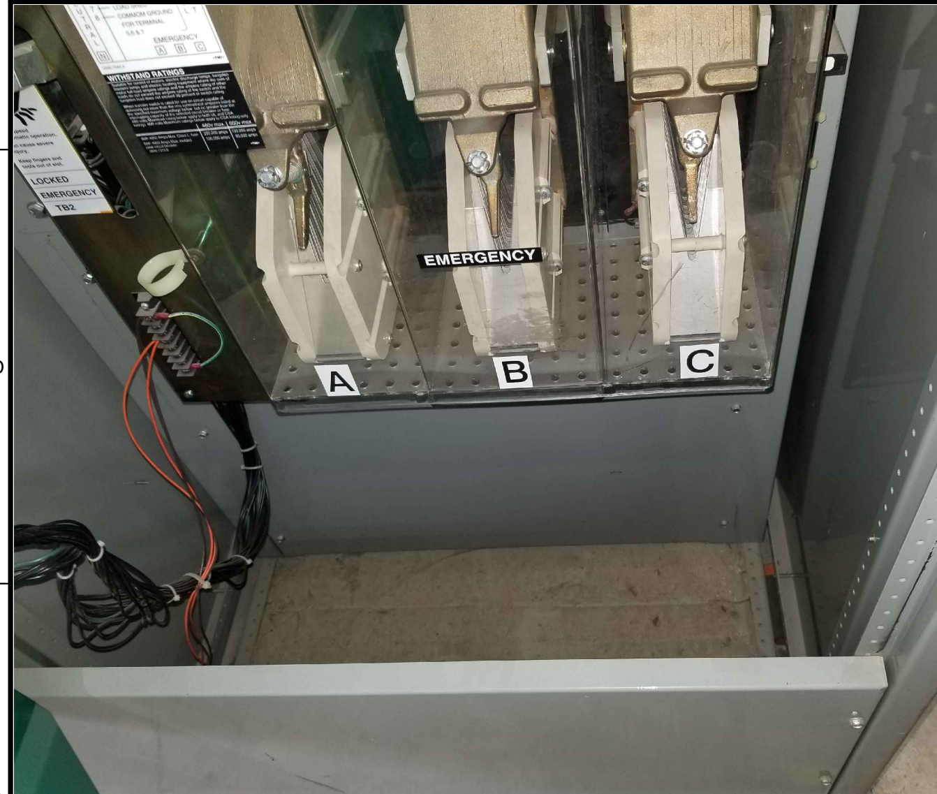
C1 PHOTO #6 - ATS - EE (EXISTING INTERIOR LOWER) DO NOT SCALE
