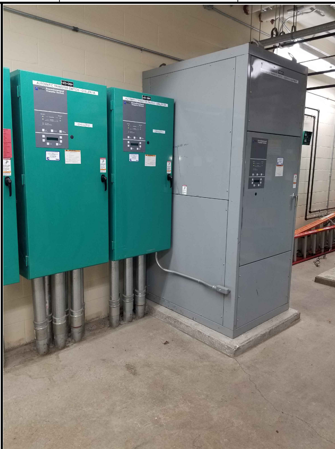
E6 PHOTO #4 - ATS - EE (EXISTING) DO NOT SCALE
