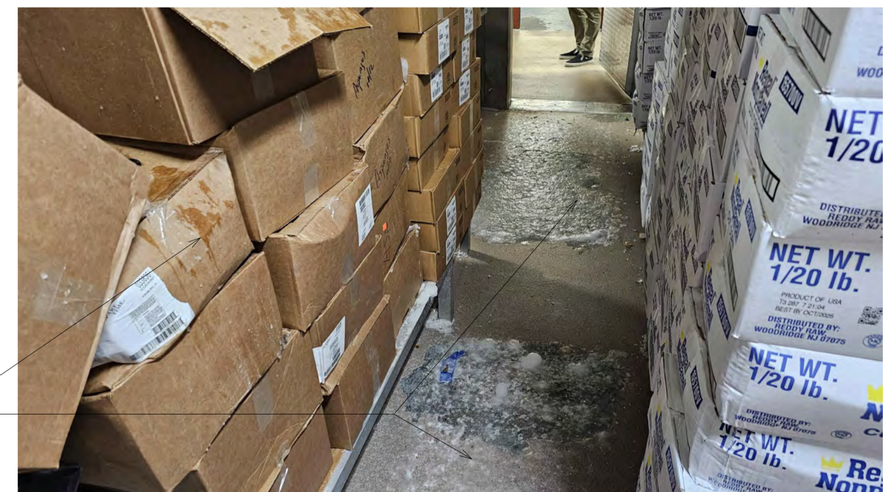
Drains around deteriorated floors may disrupt water control in the kitchen.
