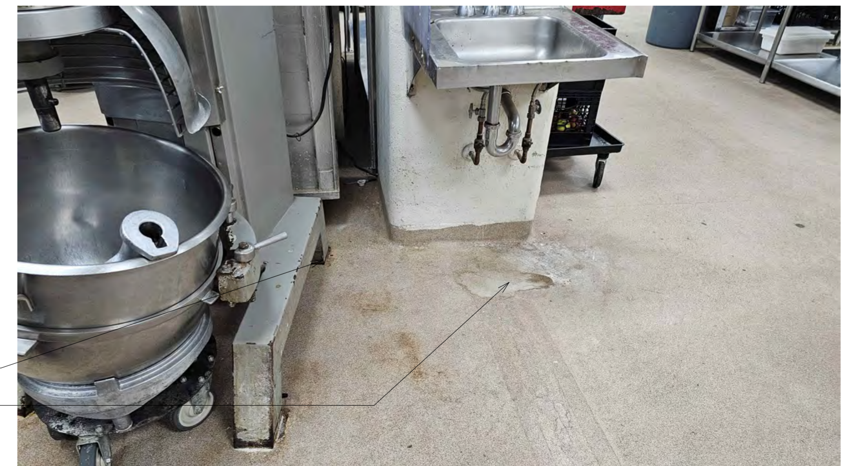
Rust from equipment rubbing into and deteriorating flooring at feet of equipment
