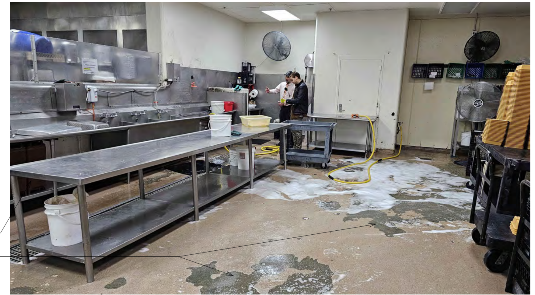
Floor deterioration @ cooking aisle, exposed aggregate of concrete below
