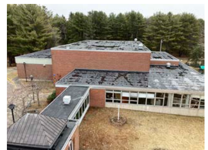
DRAPER HALL: BUILDING J
