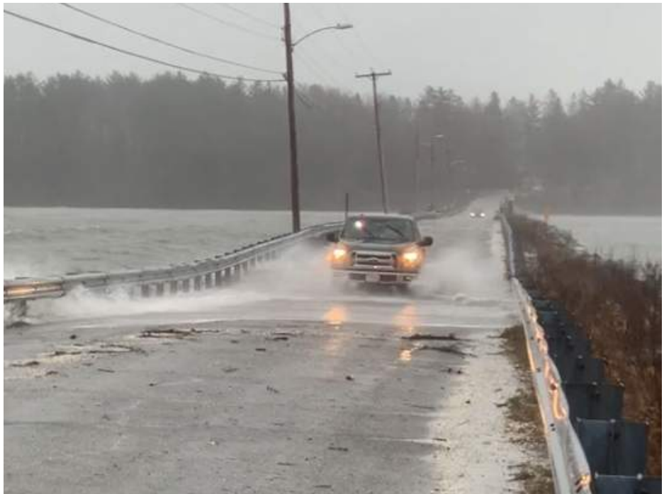
CAUSEWAY OVERTOPPING DURING DECEMBER 23, 2022 STORM
