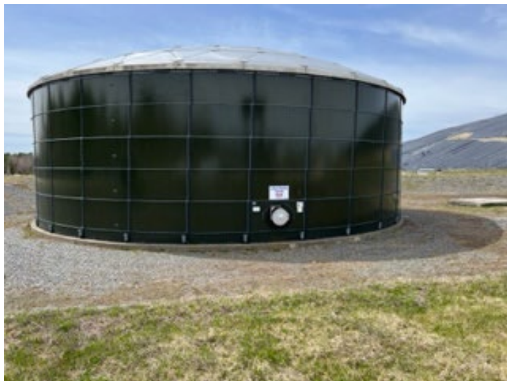
Leachate Storage Tank
