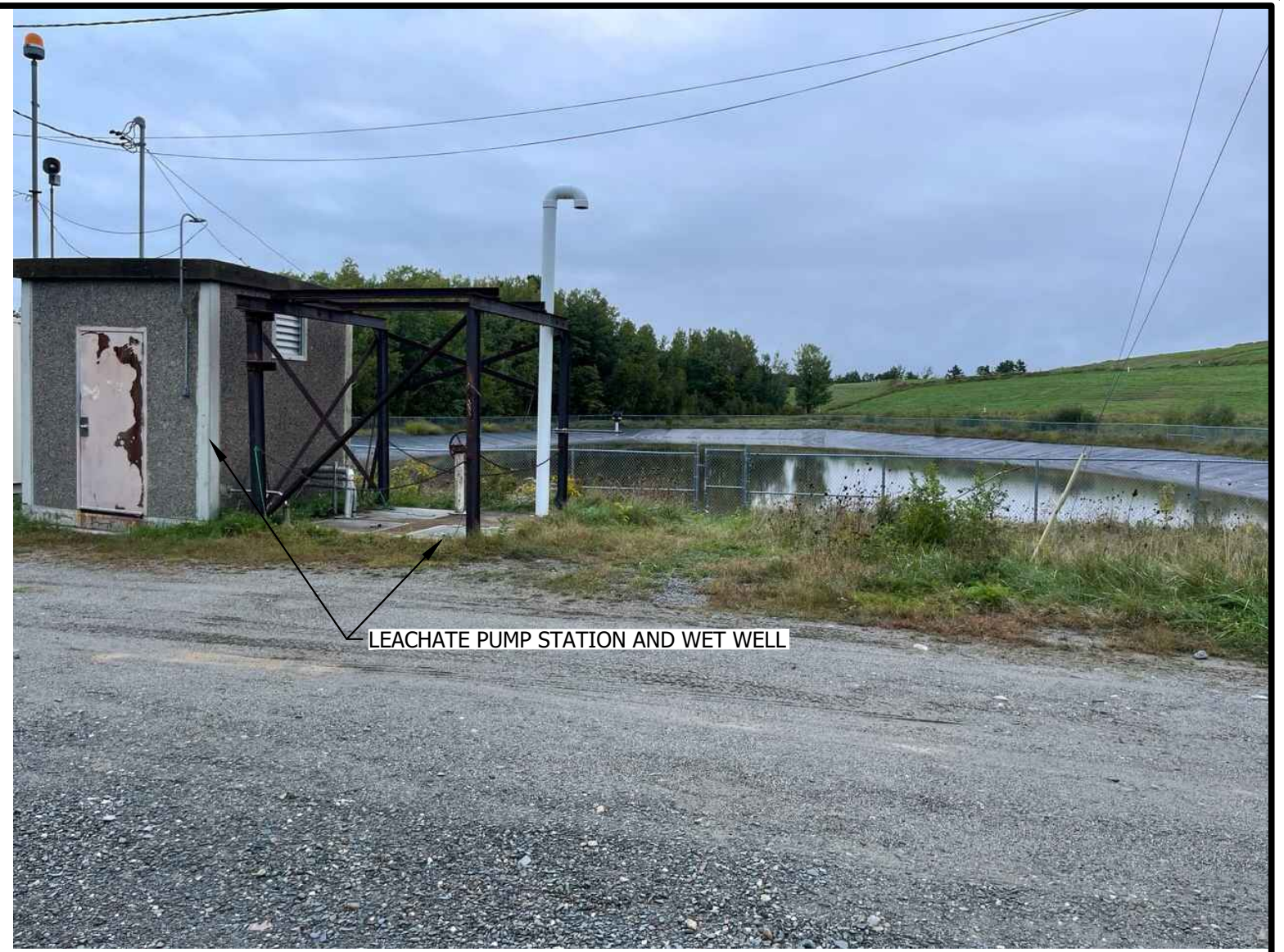
LEACHATE PIPED 3.7 MILES TO TREATMENT PLANT EMWWTP LEACHATE POND AND PUMP STATION
