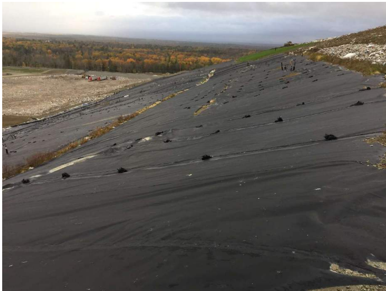
2. looking easterly across middle portion of northern slope
