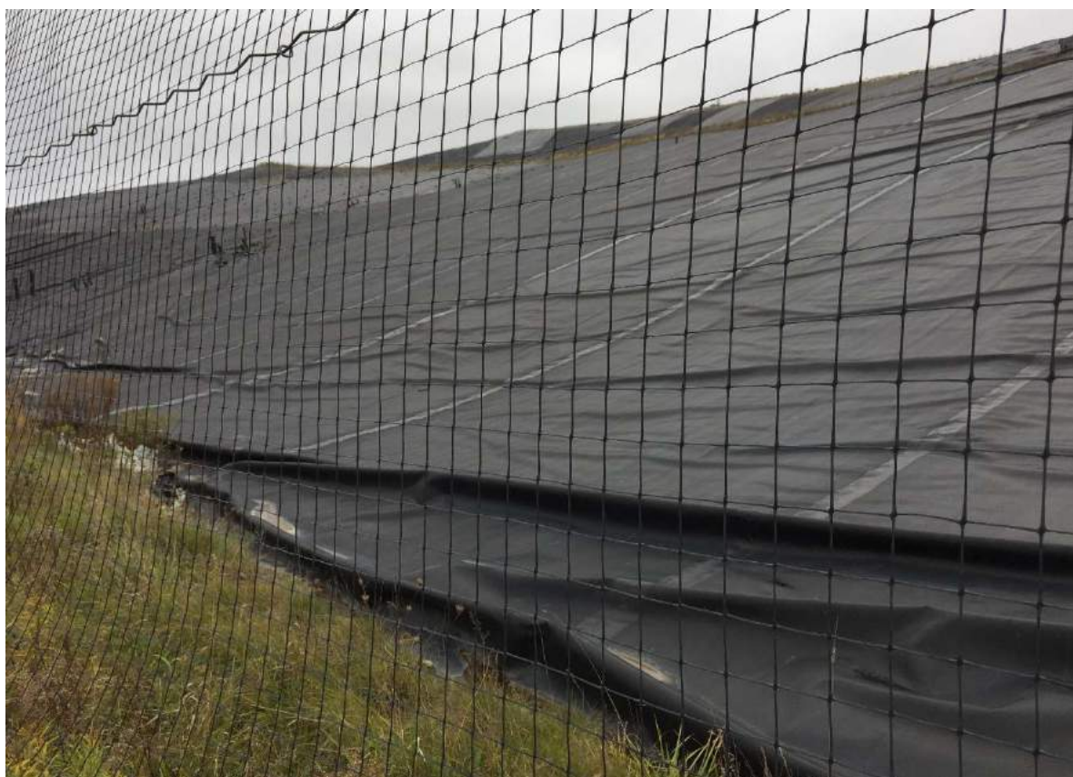
14. looking southwest along southerly slopes of Cells 4/5/6
