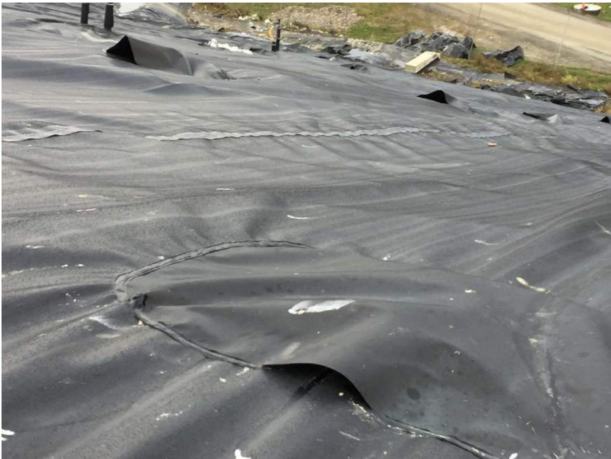
22. detail of anchor pockets on south slope of Cell 10
