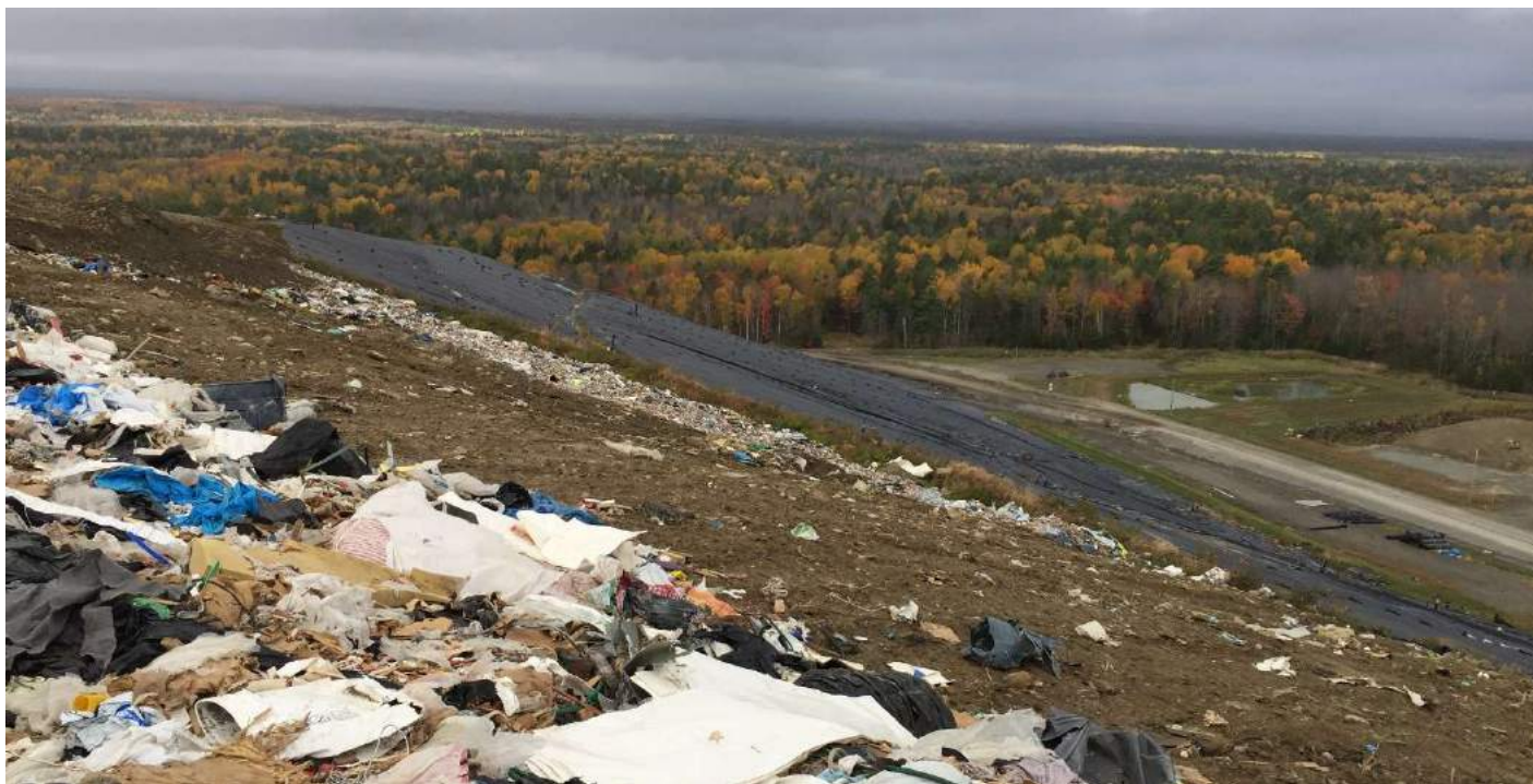
25. top of the northwest corner looking down north slope of Cell 3/2/1
