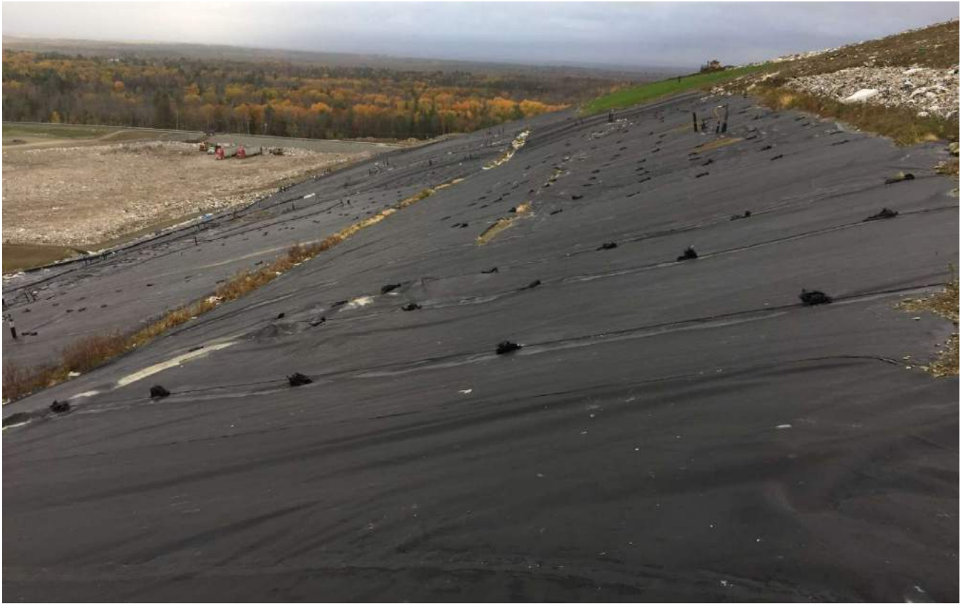
27. looking easterly along eastern north face of Cell 7/11 (with Cell 12 to the left)
