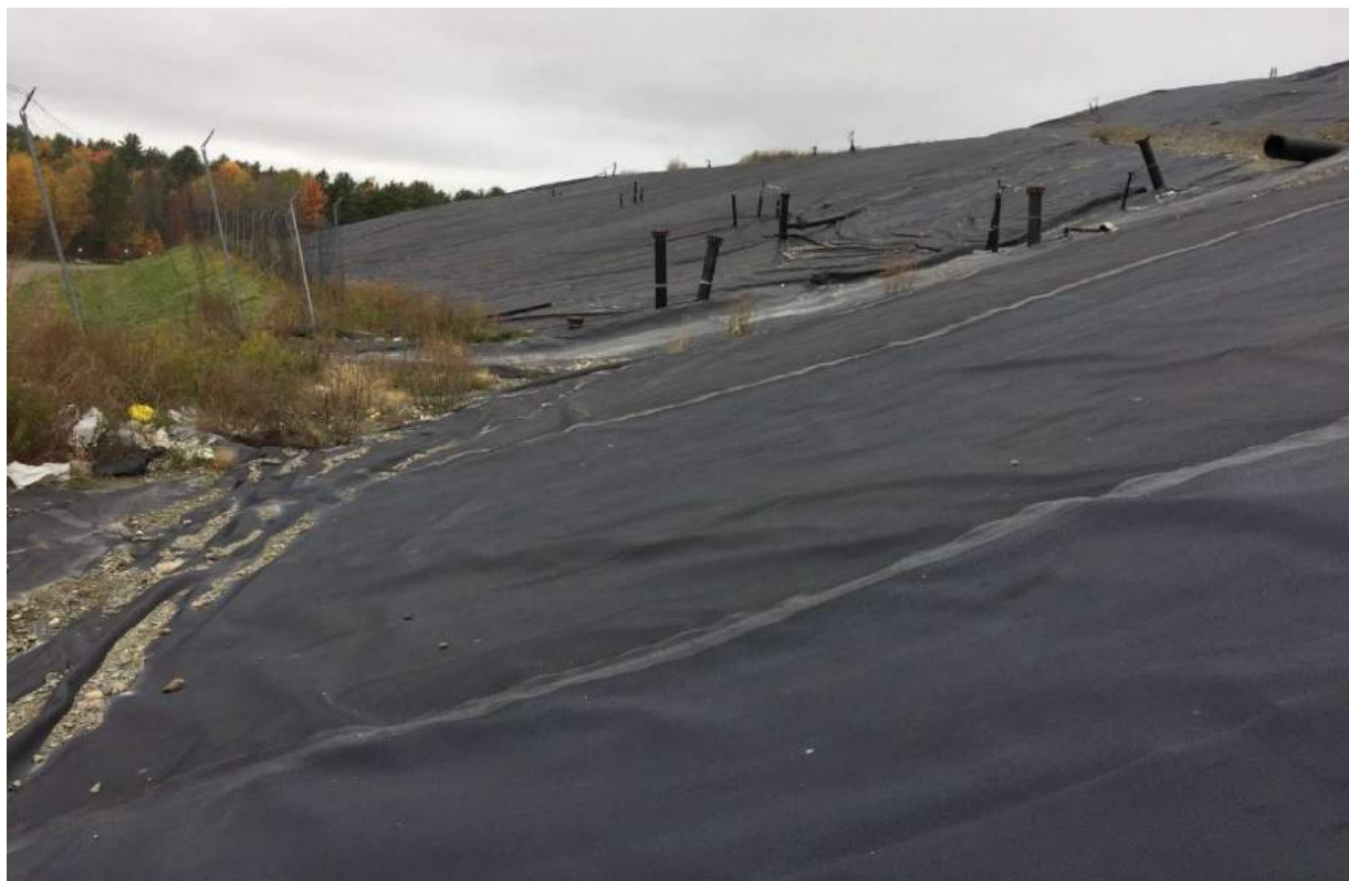
16. looking southwesterly along the bottom slope of Cell 8/10
