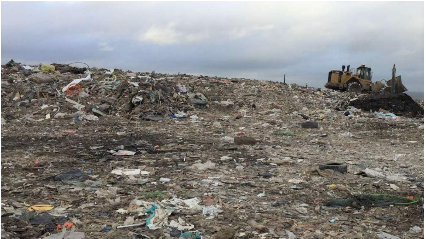
19. top of Cell 10 looking northerly to the active face of waste placement
