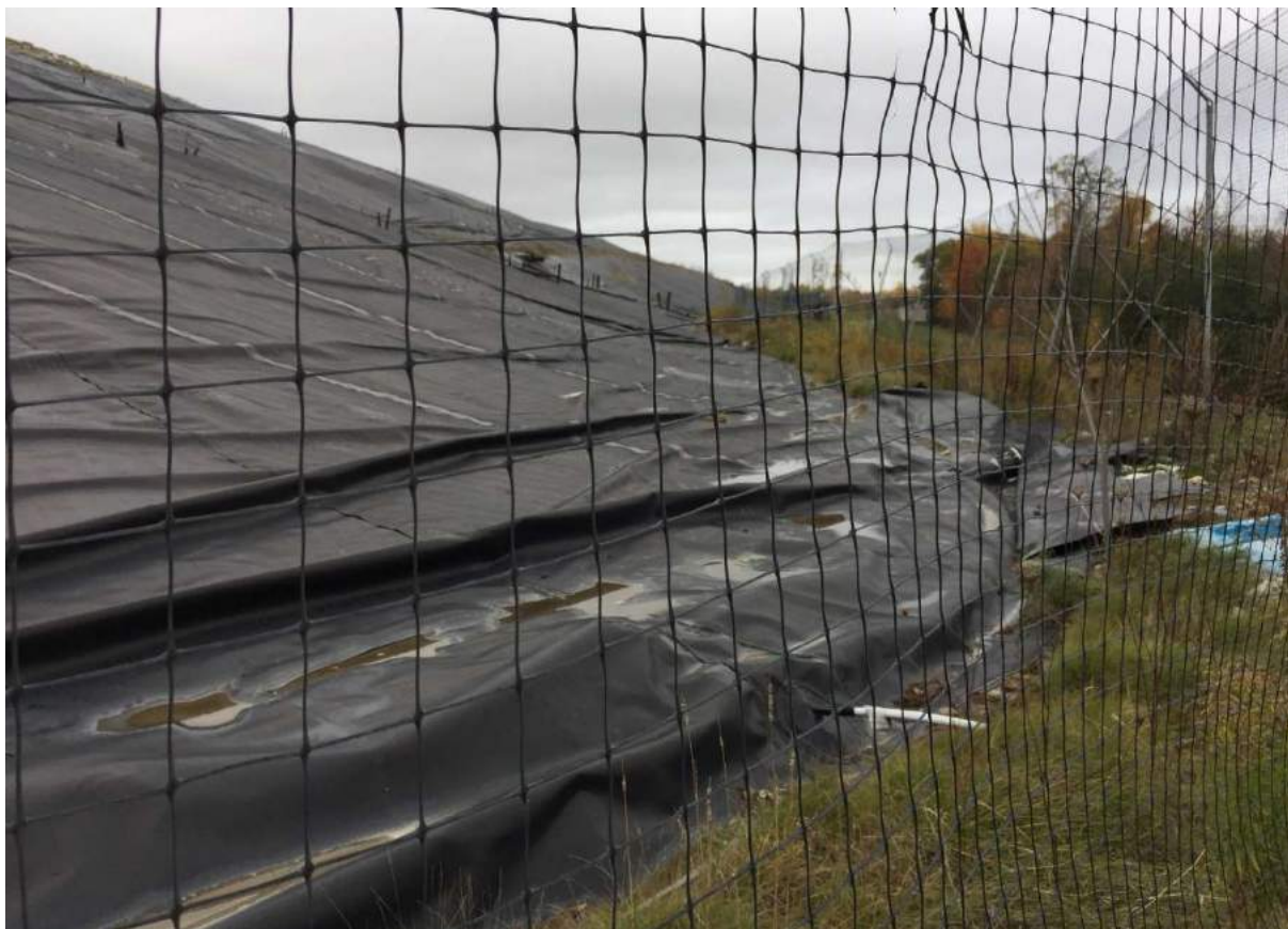
15. looking southeast to southwestern face of Cell 5/6 and Cell 8
