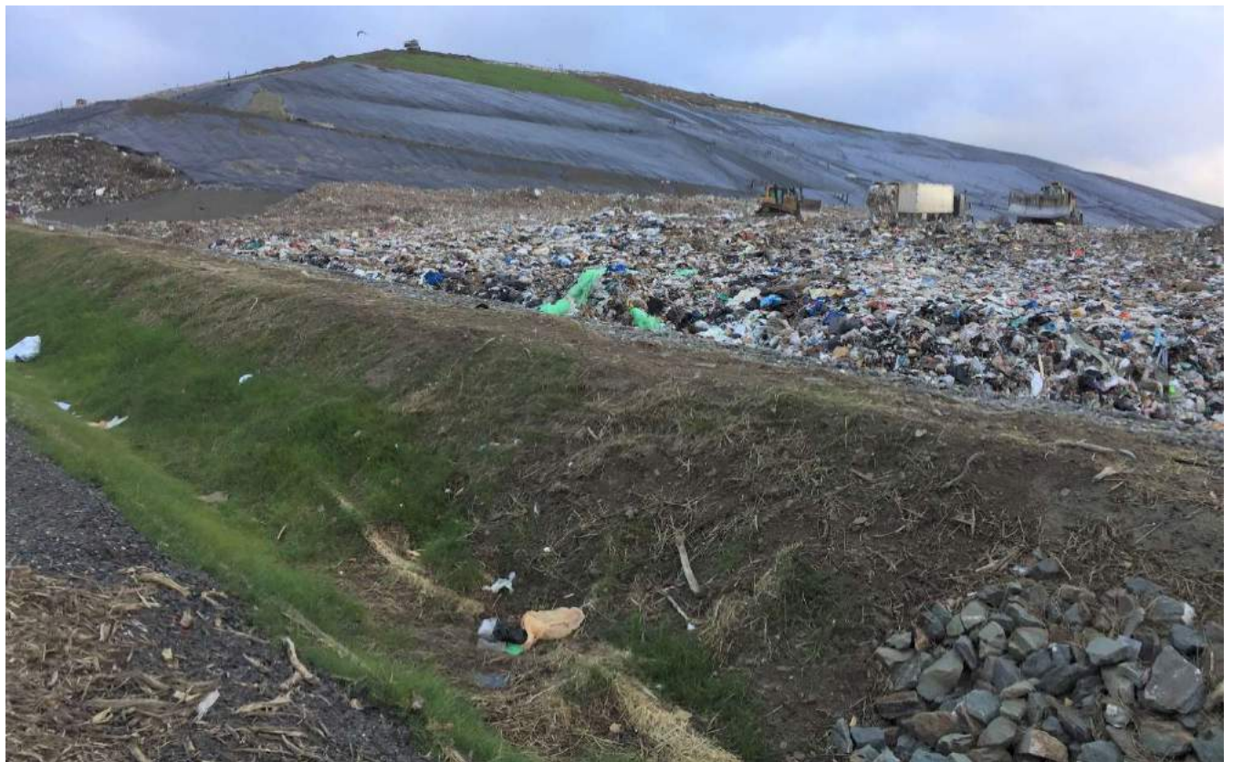
28. looking southerly towards the northeast corner of Cell 10/11 and southeast corner of Cell 12 (with the active placement of soft material in the foreground)
