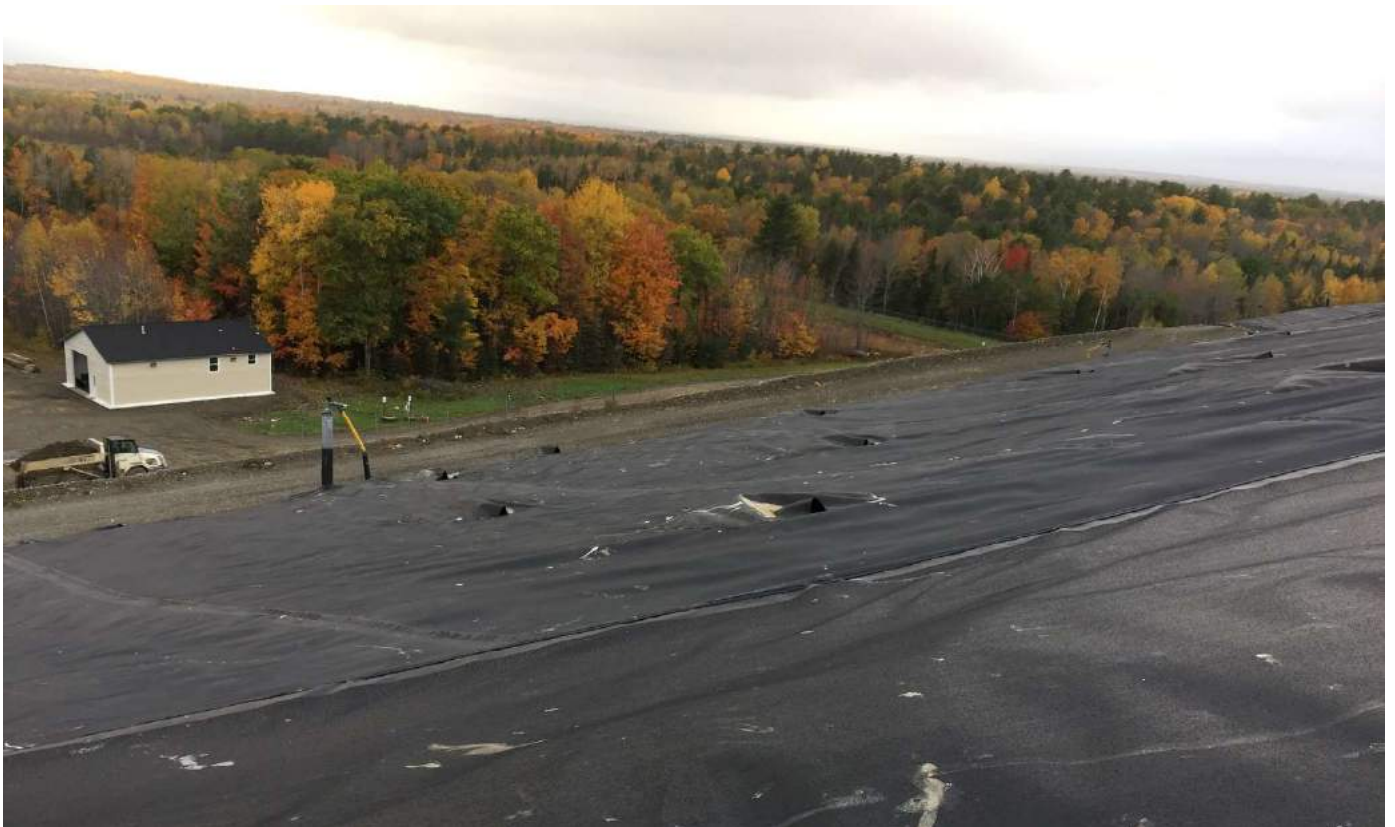
20. looking south down south slope of Cell 10
