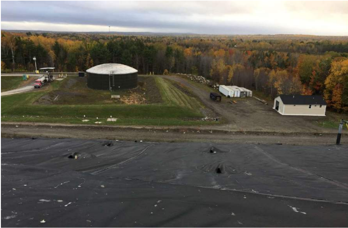
21. looking south down the south slope of Cell 10
