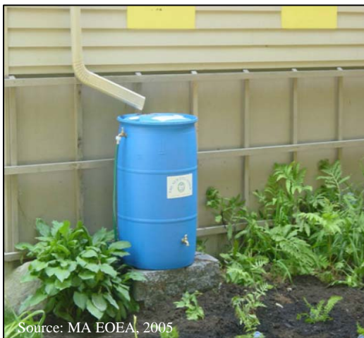
Figure 1. Residential rain barrel
