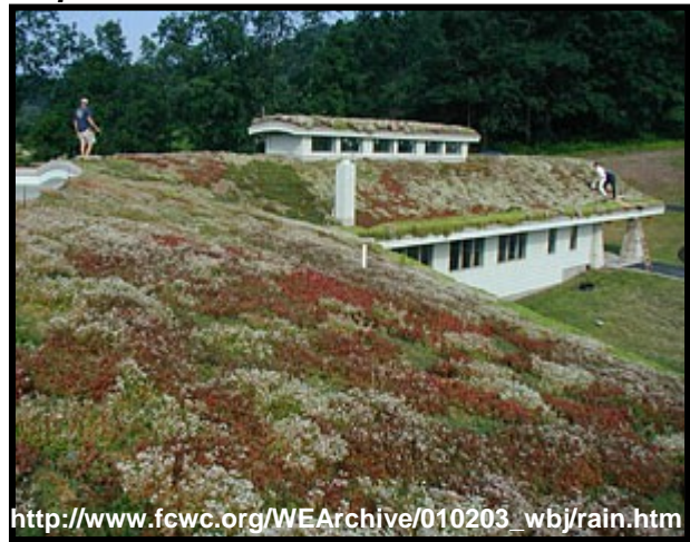
Figure 2: Green roof installed on a sloped roof
