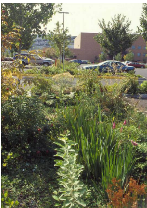
Figure 1: Vegetated Filter Strip
