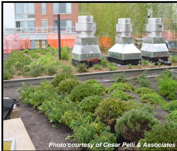
Figure 3: Green roof installed on an apartment building in Manhattan.
