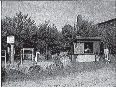
Photo C Overall view of the oil/water separator side of the system
