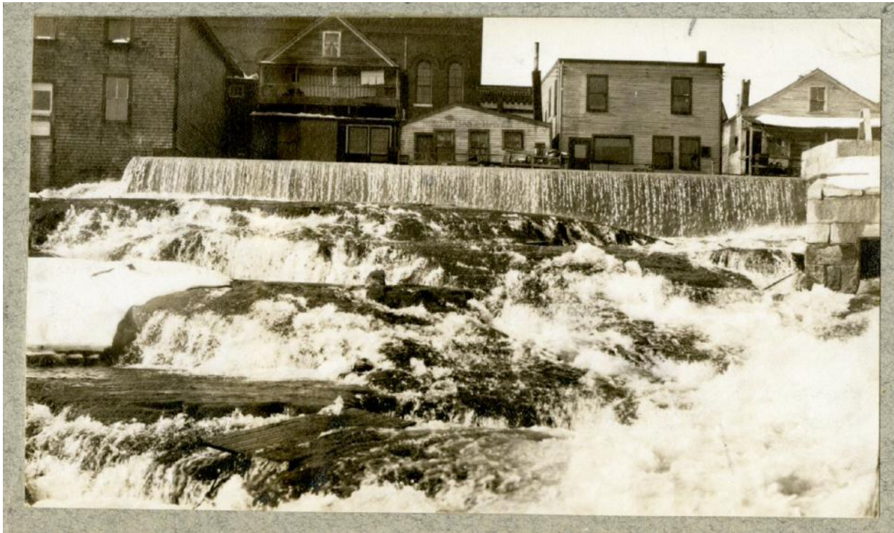
Original design by Olmsted showing the infinity pool spillway of Montgomery Dam (then called the Camden Shore Front Project) where the water level was set at 23.66 feet above sea level. Photo by Walter Clarke, January, 1931 courtesy of the National Park Service, Olmsted Archives, Frederick Law Olmsted National Historic Site, Brookline, Massachusetts.
