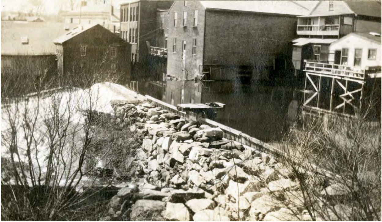
Photo of pre-Olmsted construction, courtesy of the National Park Service, Olmsted Archives, Frederick Law Olmsted National Historic Site, Brookline, Massachusetts.
