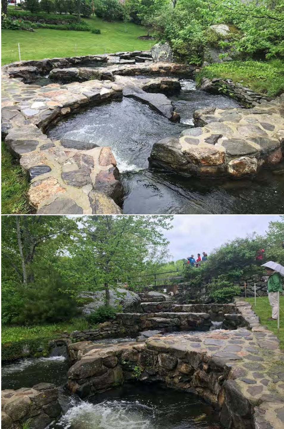
Figure 44. Pool and weir fishway at Damariscotta Mills.
