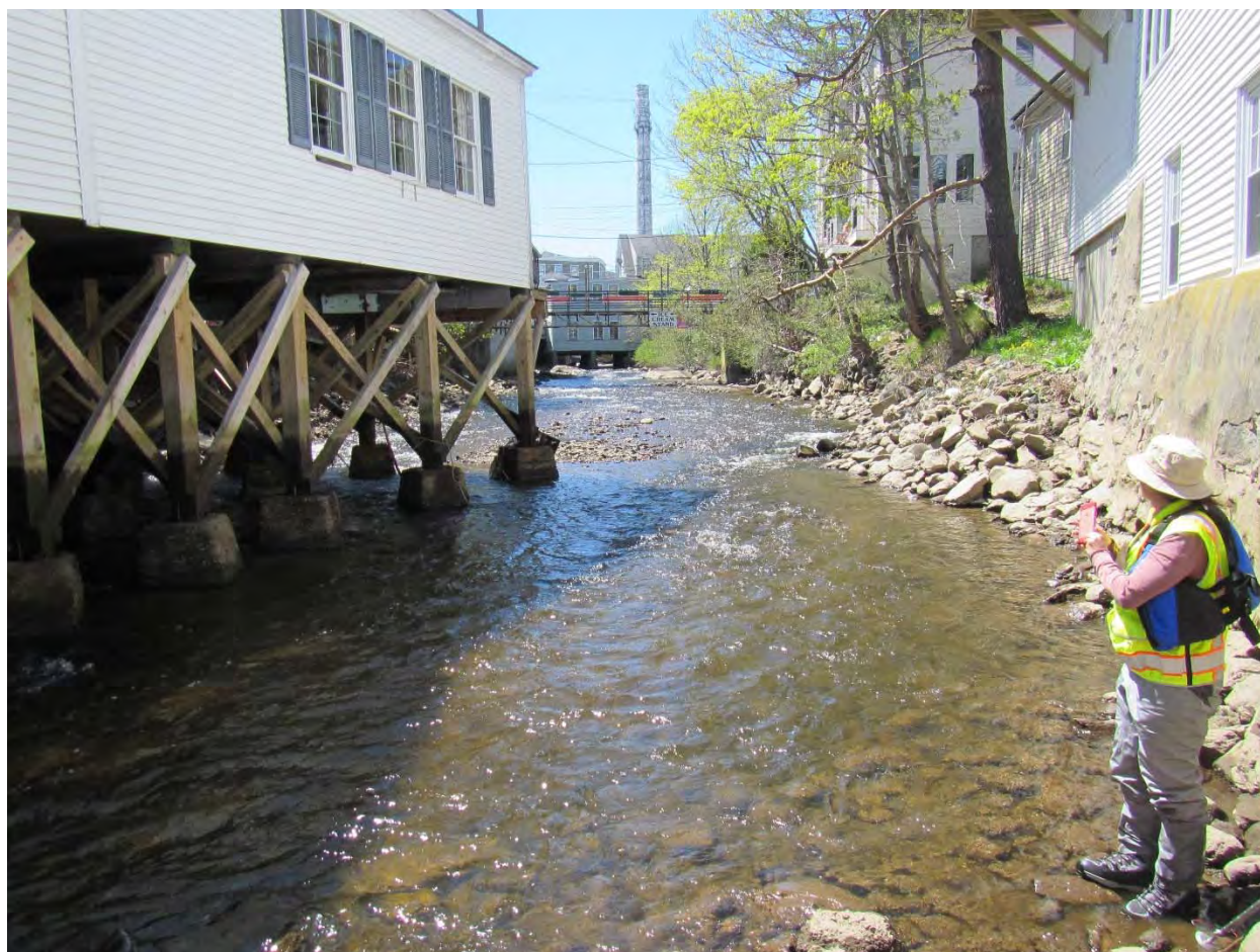
Figure 27. Looking upstream from Main Street with impoundment drawn down, May 8, 2018. In addition to infrastructure in the river, natural features such as boulders, mid-channel bars, riffles, and pools are all present through this reach.
