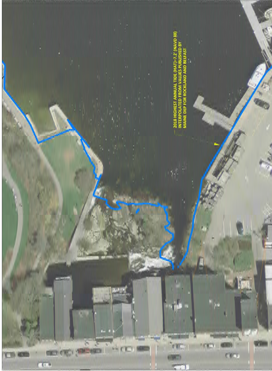
Figure 41. 2013 aerial view of Megunticook Falls and Camden Harbor showing a high tide condition (source: Maine GIS). Extreme high tides extend into the Harbor Park area over the footpath.
