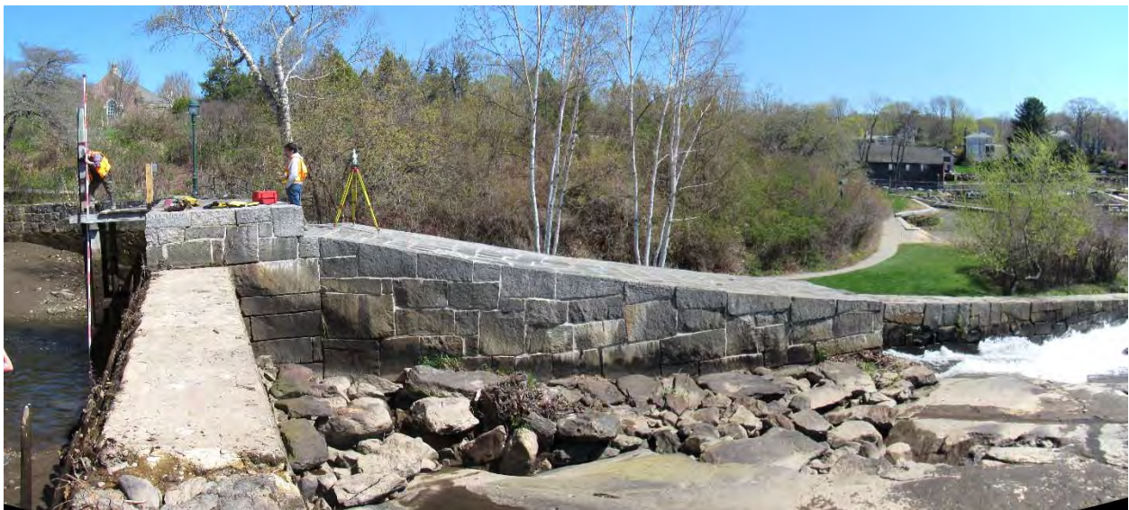
Figure 11. View of north end of spillway, the stone outflow culvert, and ledge outcrop, May 8, 2018. The seawall and Harbor Park are at the right of the image.
