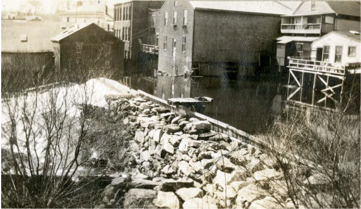
Figure 19. 1930 Photo of the dam as it existing prior to reconstruction in 1930. Photo courtesy of the National Park Service, Olmstead Archives, Frederick Law Olmsted National Historic Site, Brookline, Massachusetts.
