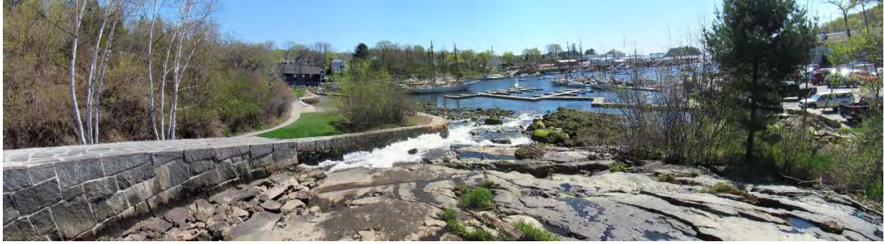
Figure 12. View east from spillway at ledge outcrop, May 8, 2018. The outflow culvert, seawall and Harbor Park are at the left of the image.
