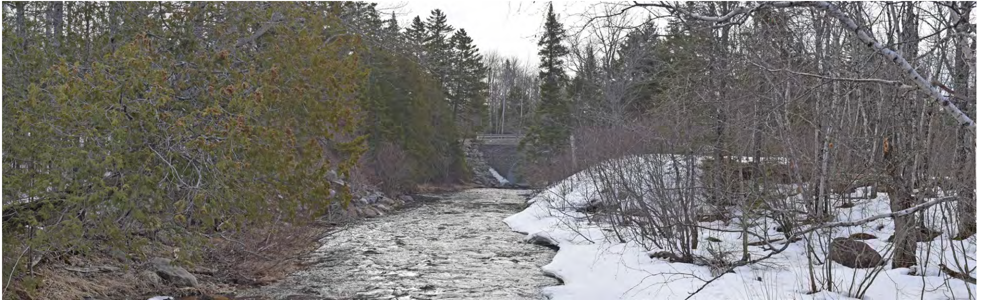
Photograph 19: Panoramic view looking east from the ITS 87 bridge over Cold Stream. The Capital Road bridge over Cold Stream is visible in the distance. The 150 foot wide proposed HVDC corridor will be visible crossing perpendicular to Cold Stream approximately 145 feet to the east. Conductors will be visible crossing the stream from this viewpoint.
