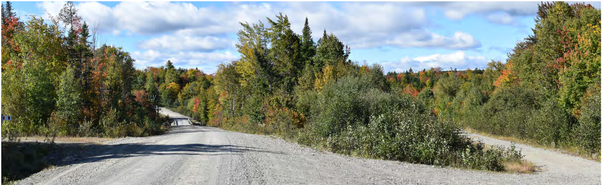
Photograph 16: Panoramic view looking west on Capital Road toward the bridge over Cold Stream. The ITS 87 bridge over Cold Stream is visible 325 feet from this viewpoint. The 150 foot wide proposed HVDC corridor will be visible paralleling the road on the right hand side of the image. Two to three structures will be visible and the closest will be approximately 80 feet from this viewpoint.
