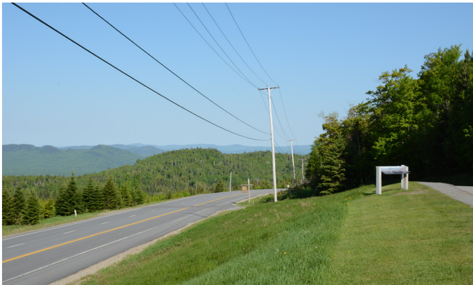
Photograph 23: View looking northwest showing the elevated rest stop above Route 201. The project will not be visible looking in this direction.
