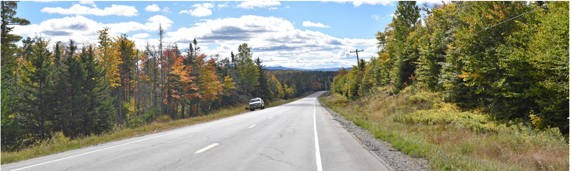
Photograph 15: View looking southeast on Route 201 in Johnson Mountain Twp from just within the proposed 150 foot wide Project corridor. The southern edge of the Project corridor is marked by orange cones in the image. Conductors will be visible above the existing distribution line. The closest proposed structures will be visible 125 feet to the east of the crossing and 800 feet to the west of the crossing.
