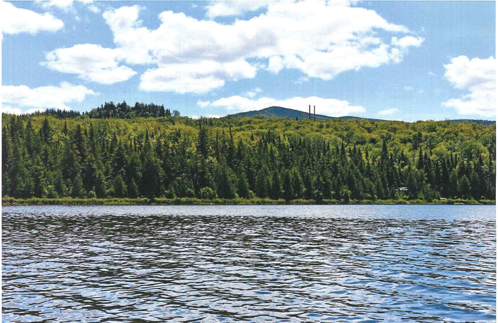
September 2017 Proposed Conditions: Normal view looking south from Beattie Pond toward the proposed HVDC transmission line. The top of one angle structure and conductors will be visible at a distance of 1,300' +/- from this viewpoint. The original September 2017 caption incorrectly noted the distance between the closest structure and the viewpoint as 1,300 feet, but that distance is actually the approximate distance between the closest structure and the edge of the pond.
