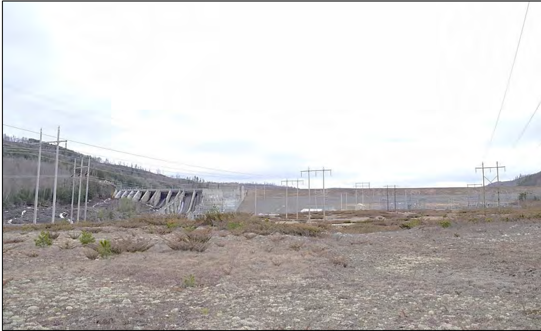
Photo 17. Wyman Dam and Powerhouse, Station Road, Moscow (Survey Map No. 428, MHPC No. 293-0001, 293-0045, 293-0047).
