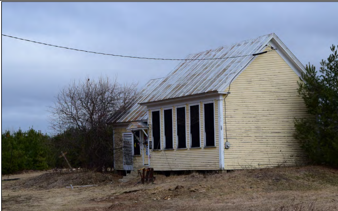
Photo 15. Former Garfield School, Kennebec River Road, Concord Twp (Survey Map No. 382, MHPC No. 534-0007).
