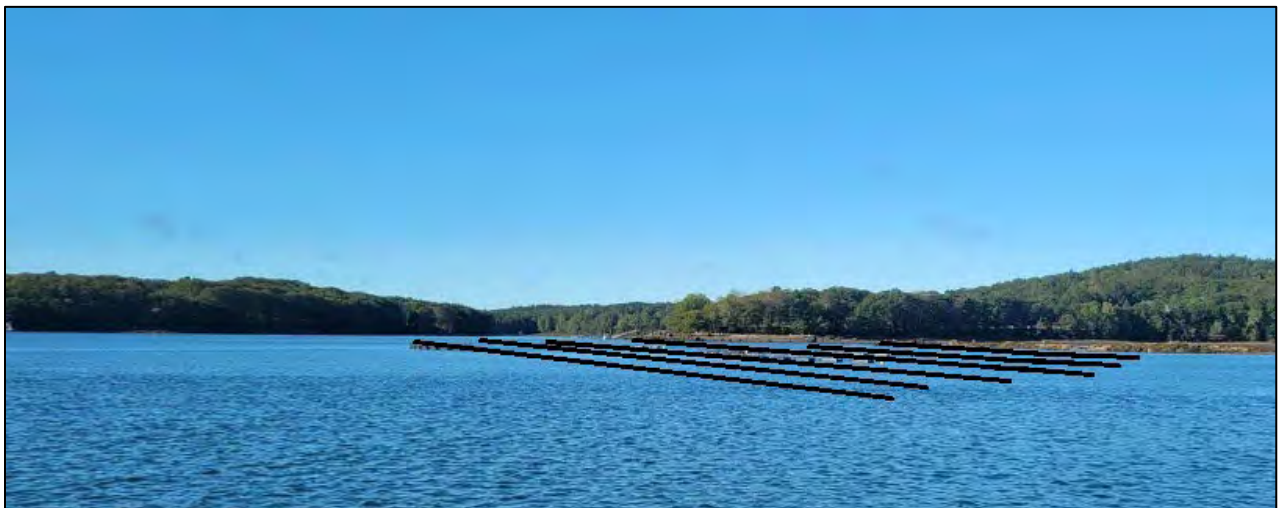
Equipment layout 2: Taken from the northeast.
