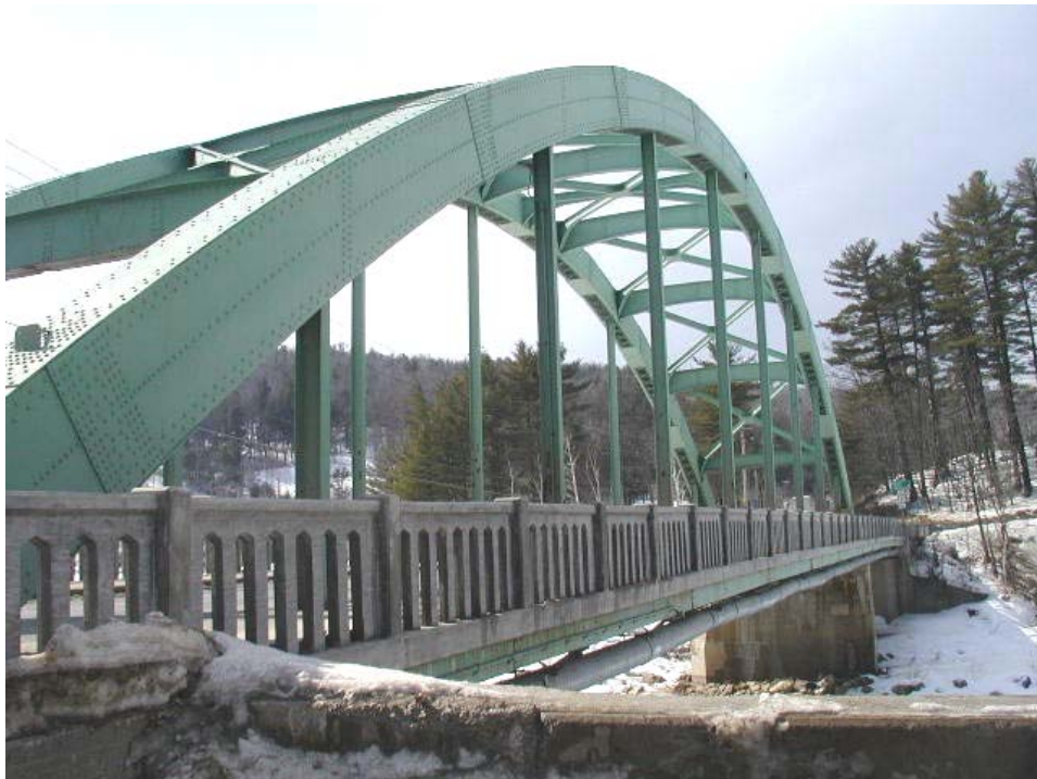
Morse Bridge, Rumford
