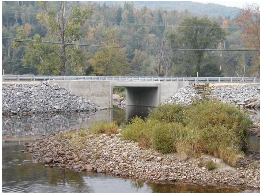
Scotty Richardson Bridge, Rumford
