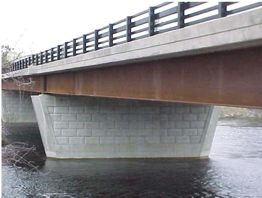
West Bridge, Fairfield-Benton
