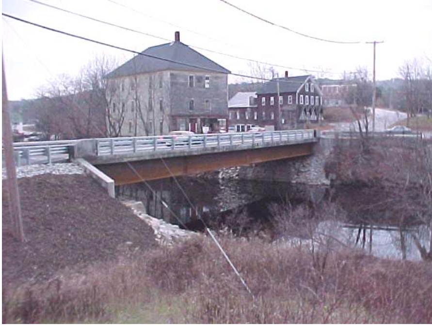
Turner Bridge, Turner
