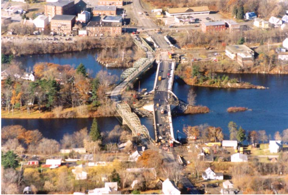
East, Center, and West Bridges, Fairfield-Benton
