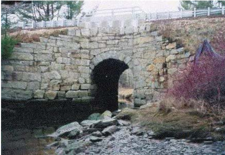
Mill Creek Bridge, Falmouth
