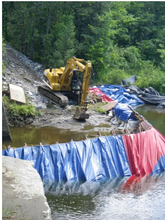
Work behind a Portadam® cofferdam.
