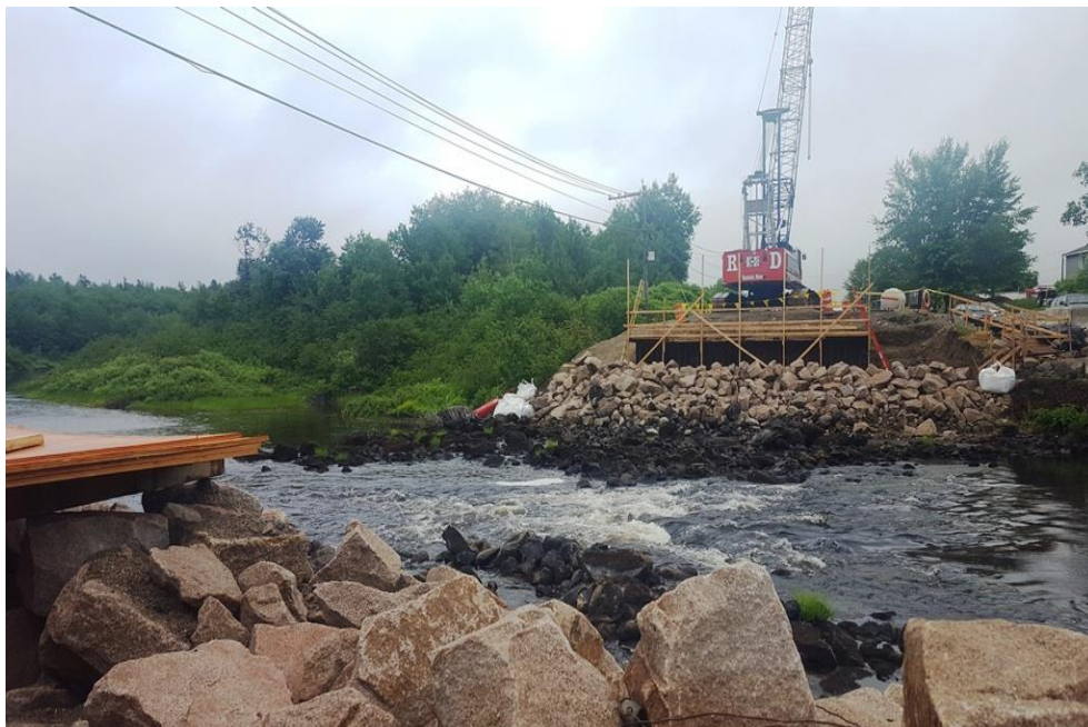
Integral Abutment Bridge During Construction
