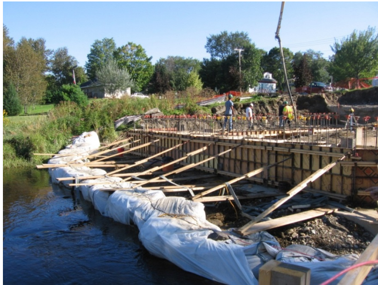
Bridge abutment construction behind a cofferdam constructed of industrial sandbags
