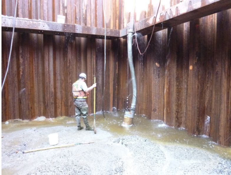
Maintenance water pumping inside sheet pile cofferdam.
