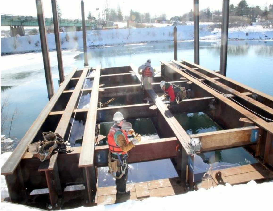
Example of a temporary work trestle being constructed
