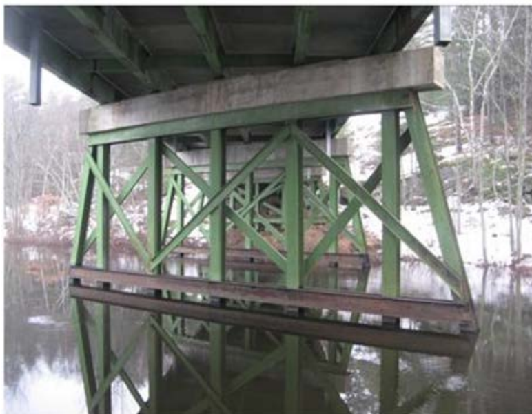
Steel pile bent showing battered piles and concrete cap
