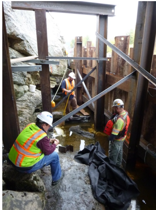
Example of the inside of a sheetpile cofferdam with extensive bracing.
