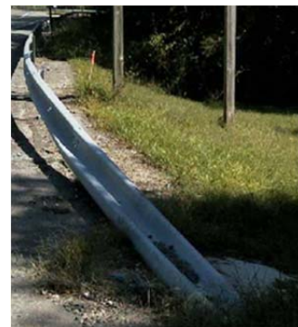
Figure 3 - Typical Turndown Installation
