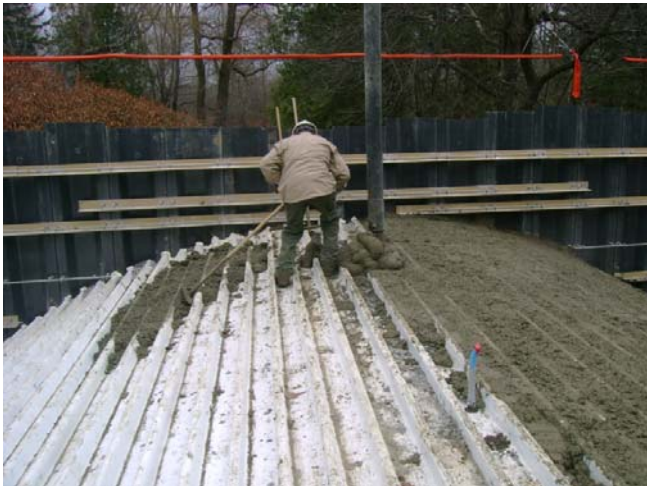
Figure 5 - Concrete placement
