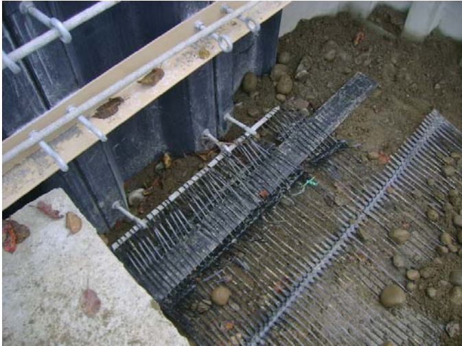
Figure 4 - MSE Retaining wall
