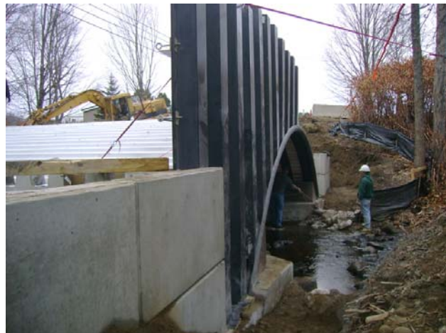
Figure 3 - Installation of composite retaining wall
