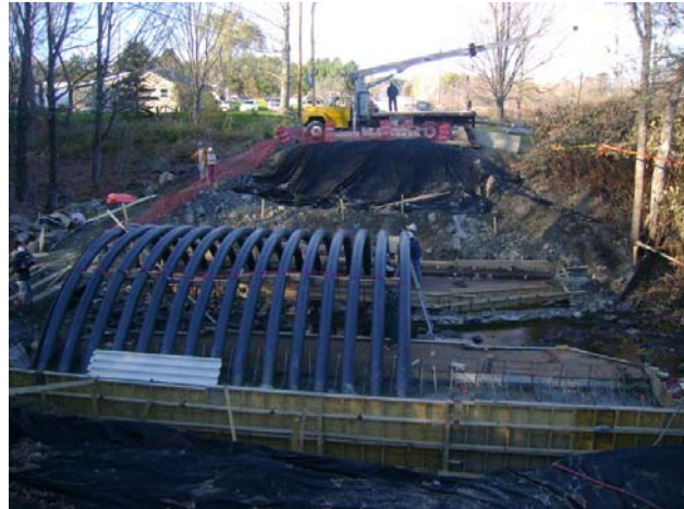
Figure 1 - Installing Composite Arches
