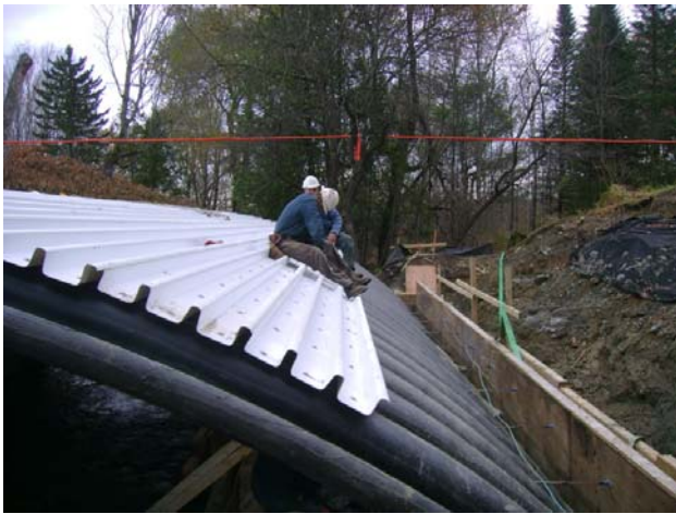
Figure 2 - Installing composite decking
