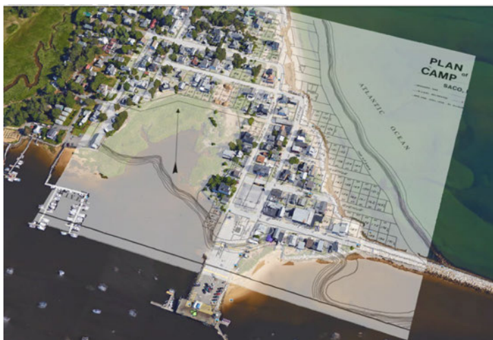
Figure 3.40: (Left) Aerial photograph of the Saco River jetties and Camp Ellis. Incoming waves during northeast storms reflect off the northern jetty and focus wave energy along Camp Ellis Beach. Tax map overlay from 1908 indicates the number of parcels that have been lost by erosion. Erosion rates immediately adjacent to the jetty are 2-4 feet per year. A deep trough adjacent to the jetty has formed. Map created by Maine Geological Survey.
