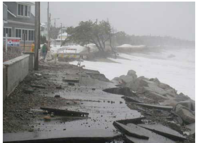
Figure 3.7: Damage from the Patriot’s Day Storm, 2007 Photo by John Cannon. National Weather
