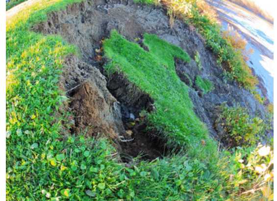
Figure 3.54: 2021 Rockport landslide. Photo courtesy of Knox County EMA.
