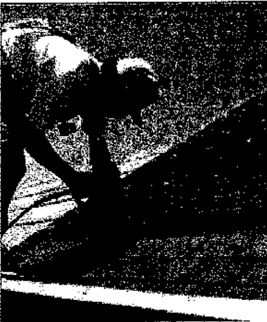
These roof shingles are coated with PV cells made of amorphous silicon. When installation is complete, the PV shingles look much like ordinary roofing shingles, but they generate electricity.
