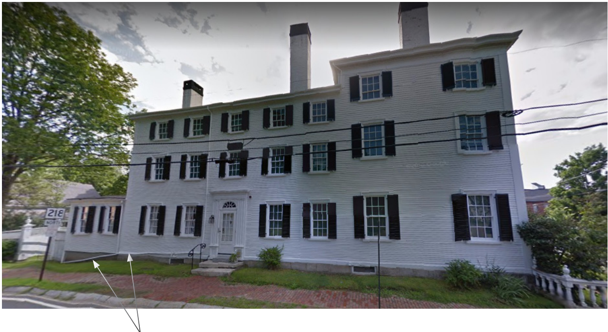
Above: At Nickels-Sortwell, runoff from the roof of the main house, the three-story ell, and the one-story ell all flow into nearly horizontal lengths of pipe. The pipe at the one-story ell is carrying the most runoff. Source: Google maps.
