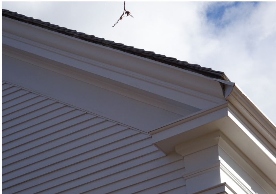
Above, the original condition of the cornice and cornice return on the Marrett House barn. As shown below, the molding at the eave was replaced with a metal gutter formed to resemble wood moldings. The profile of the gutter does not match the original molding at the rake, so the two pieces do not meet properly. Photographs taken by Margaret Gaertner, April 20, 2018.
