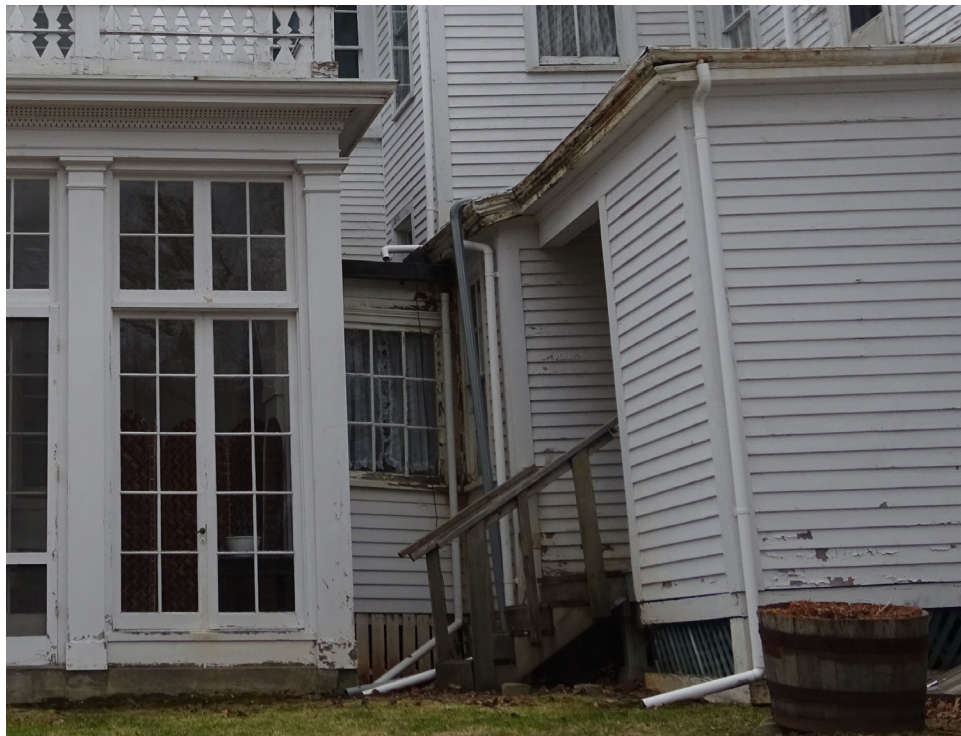
Above, the north facade of the main house and solarium. Several leaders drain into the space to the right of the solarium, causing settlement in the building, paint failure and decay of wood cornices and gutters. Below, a closer view of the decay and paint failure. Photographs taken by Margaret Gaertner, April 20, 2018.
