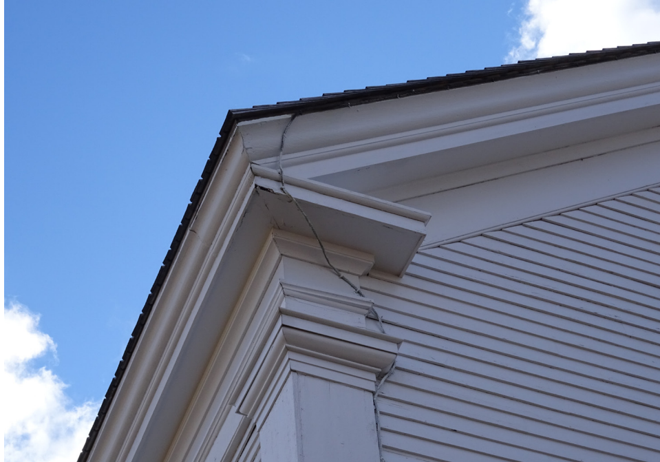
Above, the original condition of the cornice and cornice return on the Marrett House barn. As shown below, the molding at the eave was replaced with a metal gutter formed to resemble wood moldings. The profile of the gutter does not match the original molding at the rake, so the two pieces do not meet properly. Photographs taken by Margaret Gaertner, April 20, 2018.
