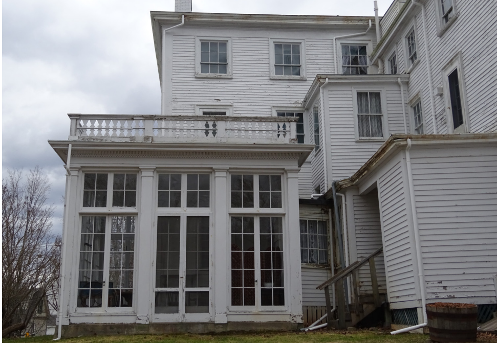
Above, the north facade of the main house and solarium. Several leaders drain into the space to the right of the solarium, causing settlement in the building, paint failure and decay of wood cornices and gutters. Below, a closer view of the decay and paint failure. Photographs taken by Margaret Gaertner, April 20, 2018.
