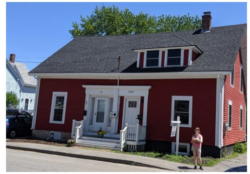
Greek Revival 148-150 Sawyer Street in Ferry Village
