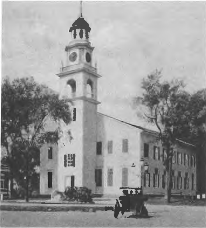
Figure 3. First Parish Church, Kennebunk, 1909 view (MHPC).
