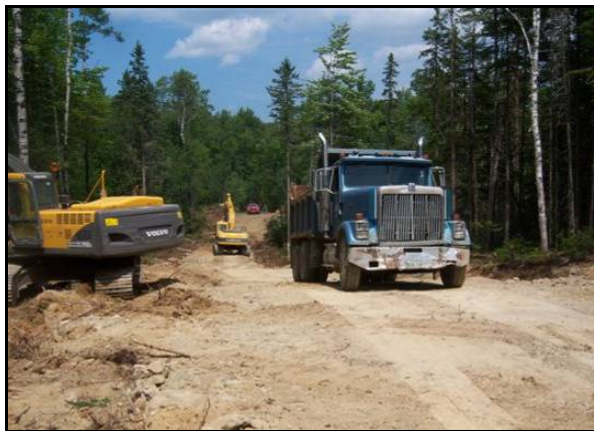
Management Road Construction at Nahmakanta
