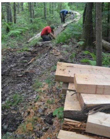
Workers from the Northern Forest Canoe Trail Installing Bog Bridging
