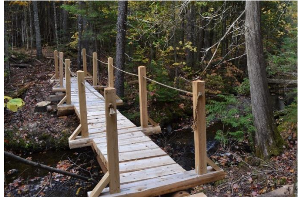
New footbridge constructed at Little Moose, in the BPL Western Region.
